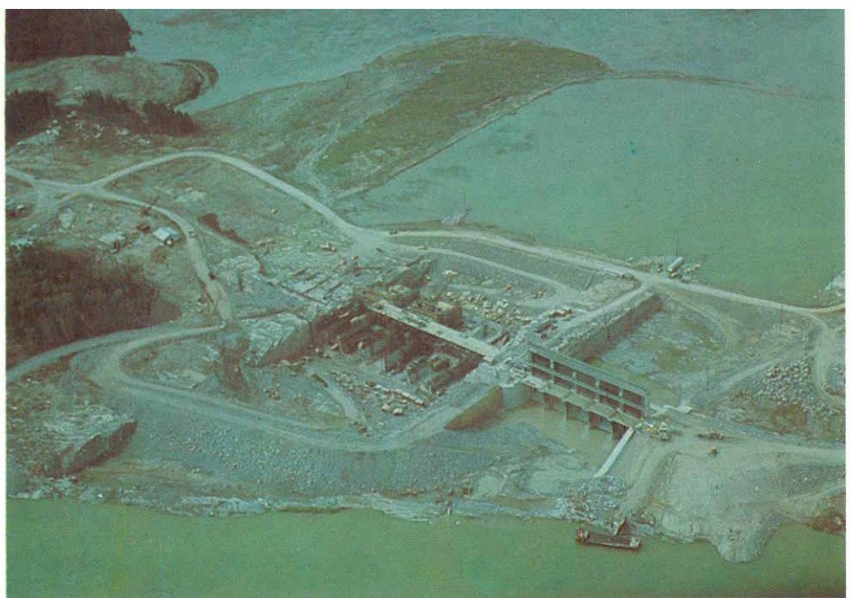
Jenpeg Construction, Summer 1974 (Study Board).
