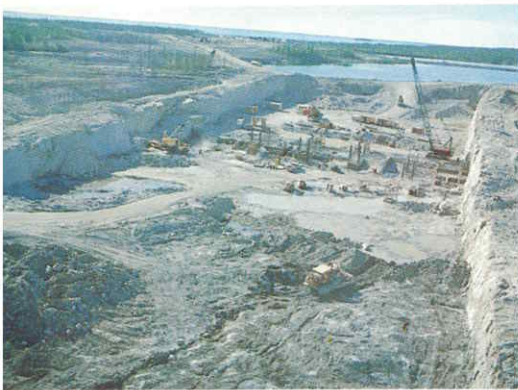
Construction at Missi Falls, Summer 1974 (Manitoba Hydro).
