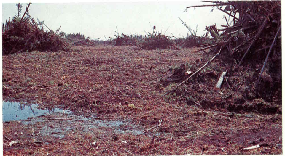
Clearing Piles, Jenpeg (R. J. Lay).
