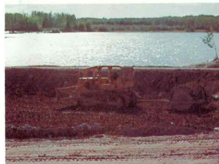
Kiskitto Dam, Construction (R. J. Lay).
