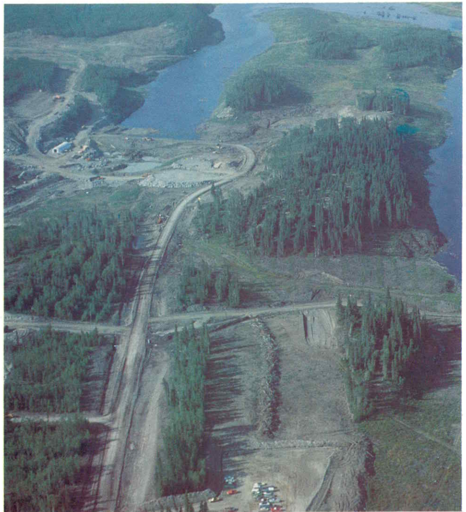
Construction Activity at Notigi (Study Board).
