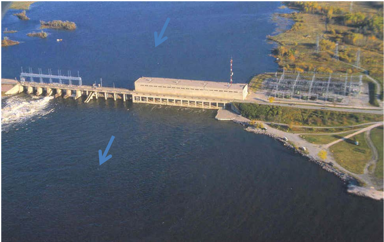
Figure 3 Pine Falls Generating Station
