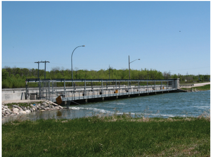
Fairford Control Structure
