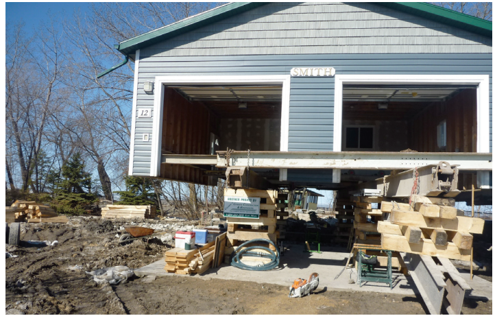
Raising permanent dwelling to higher elevation
