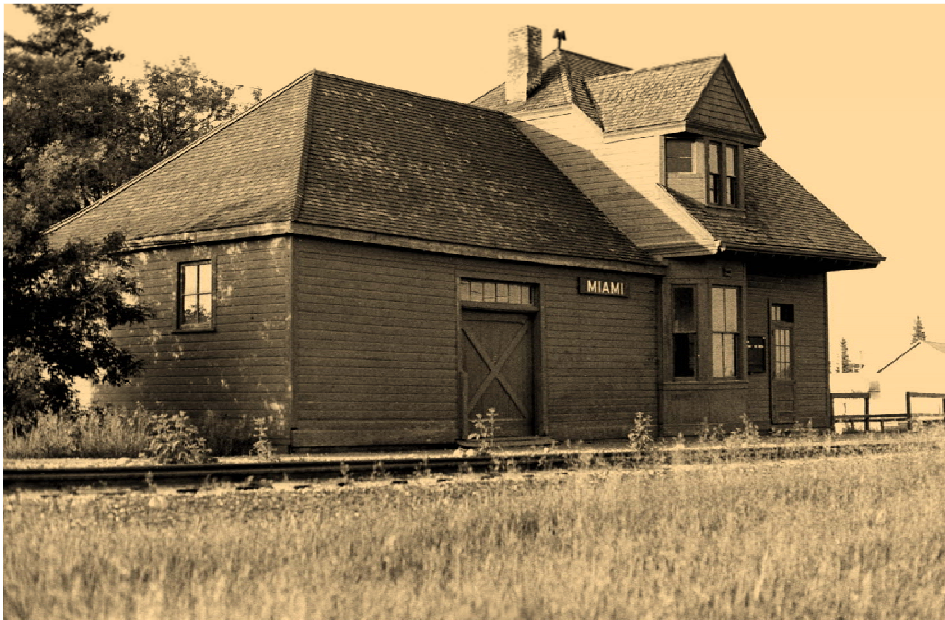
Figure 12 The Northern Pacific Station at Miami.
