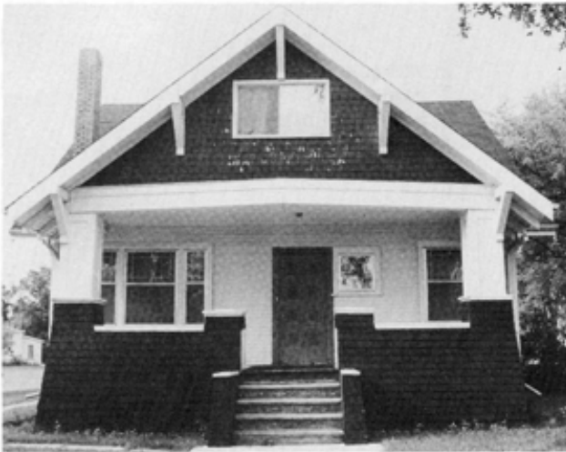
57. River Road, Arborg, 1914. Typical of the style, the outdoor space of the verandah is enclosed within the body of the house.
