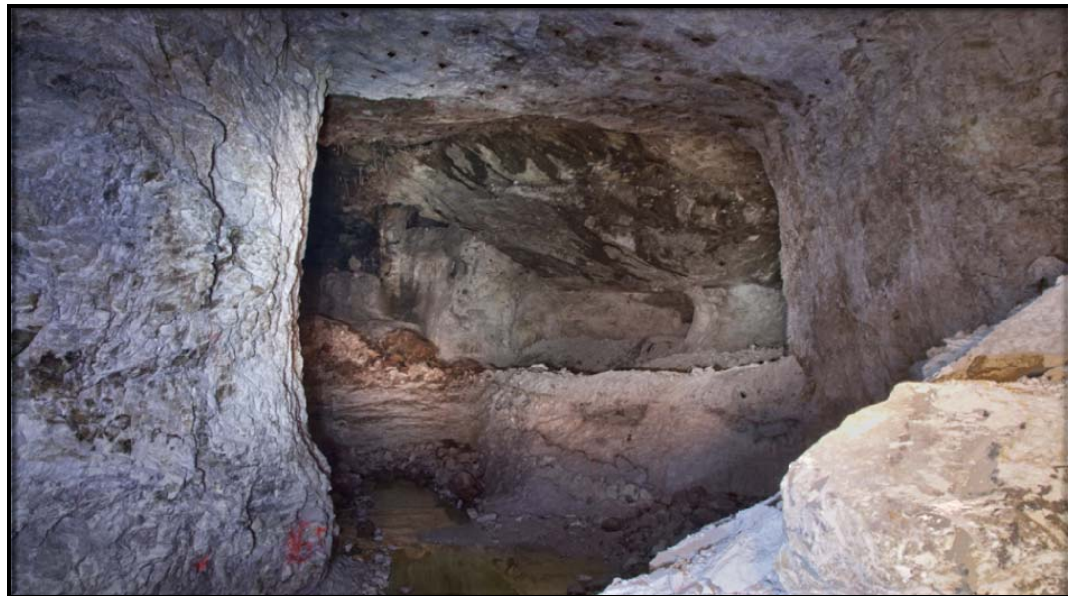
Figure 2.1 Underground Picture of the Affected Roof
