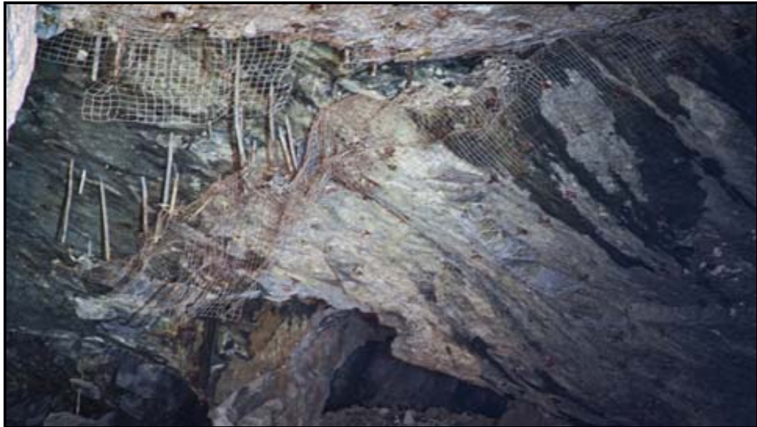
Figure 2.4 Close-up Picture Showing Condition of the Failure Zone
