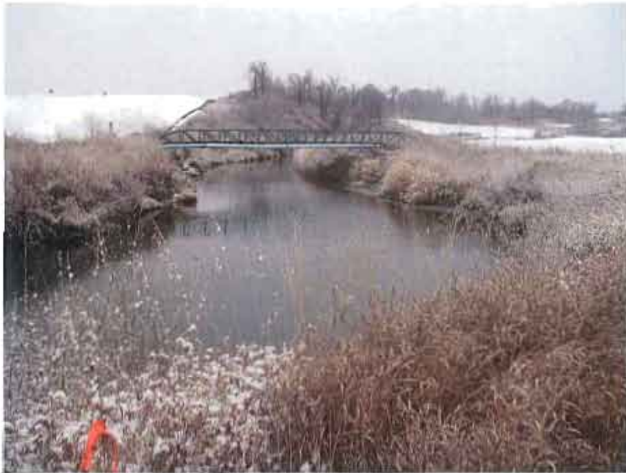
Photograph No. 6: Cross-section 6.
