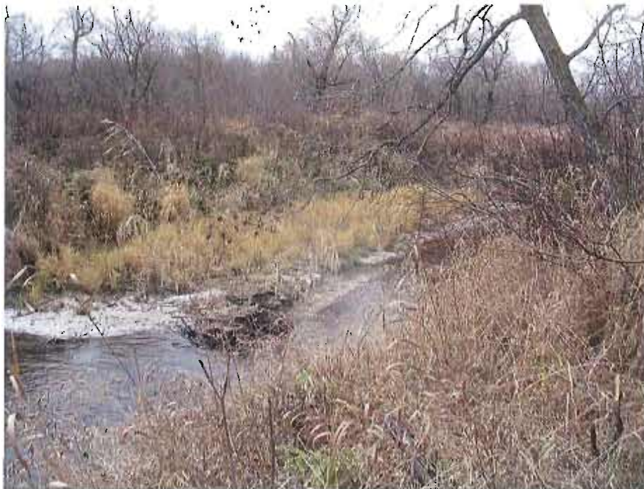
Photograph No. 12: Cross-section 12.
