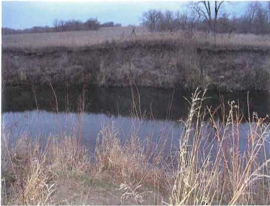
Photograph No. 11: Cross-section 11.
