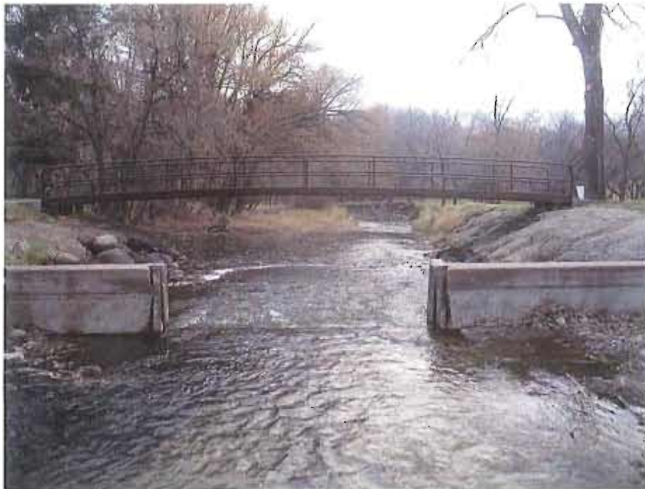
Photograph No. 1: Cross-section 1 Control Structure.
