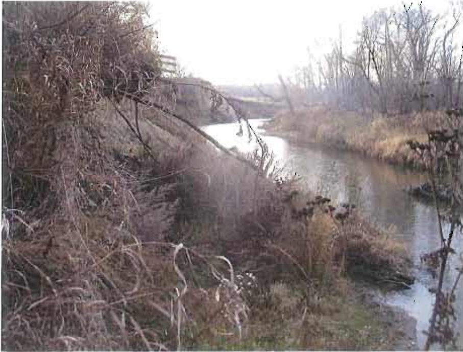
Photograph No. 15: Cross-section 17.
