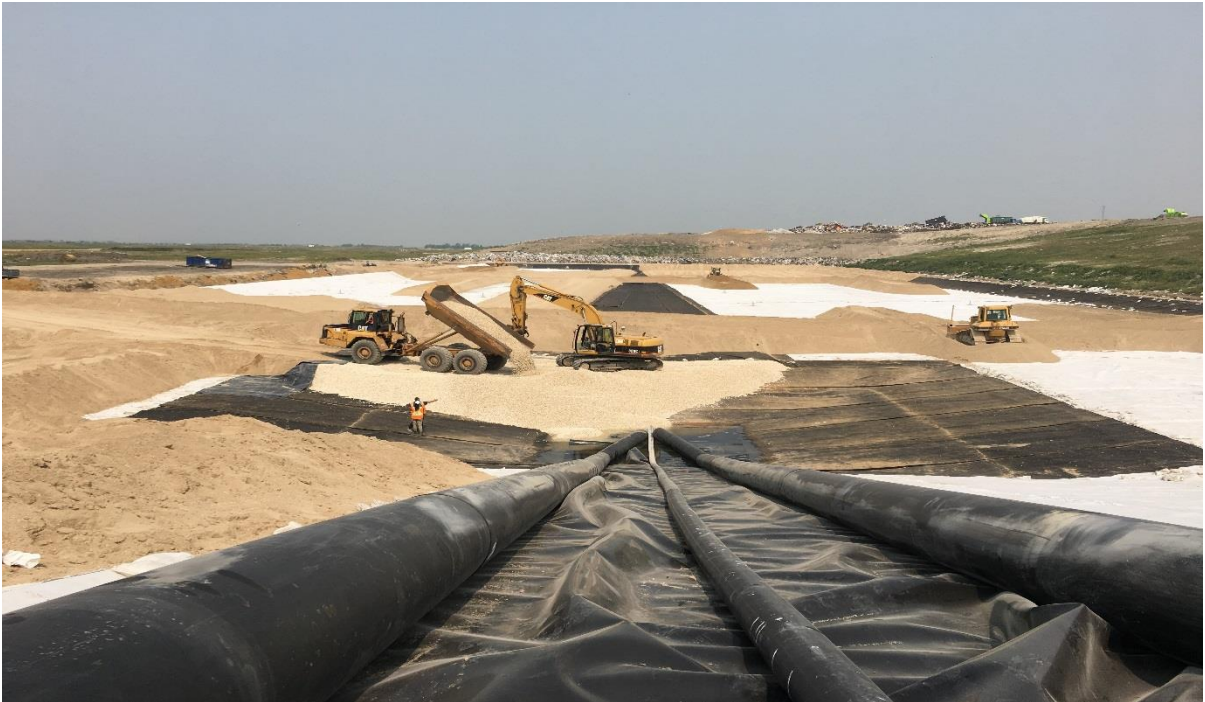
Installation of Leachate Collection 50 mm clean stone in sump
