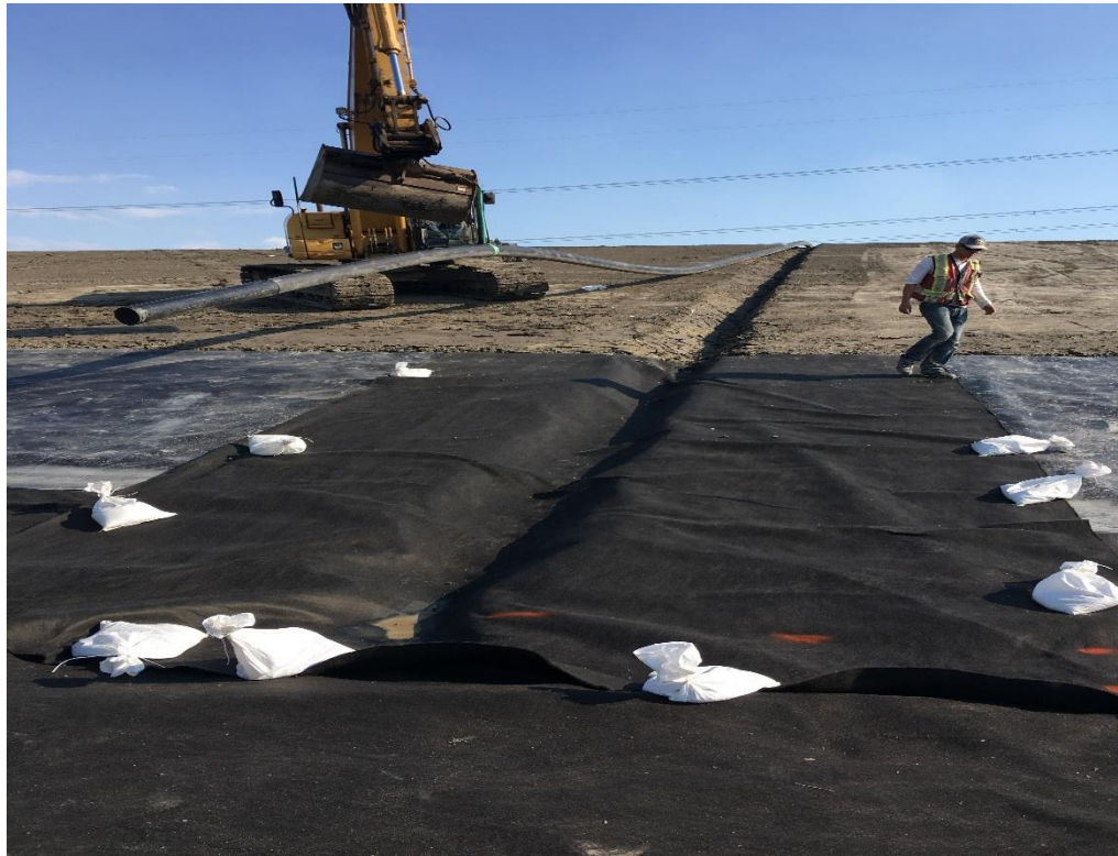
Installation of Subliner Sampler Pipe
