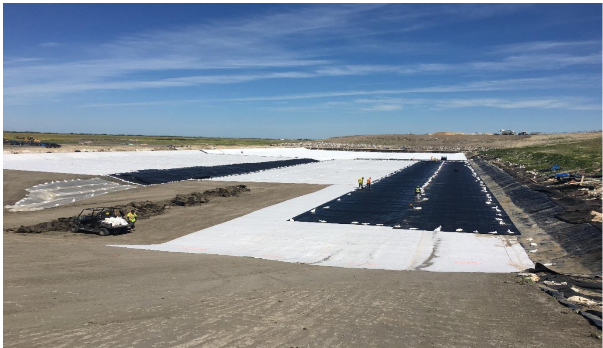
HDPE deployment and tie into Cell 13
