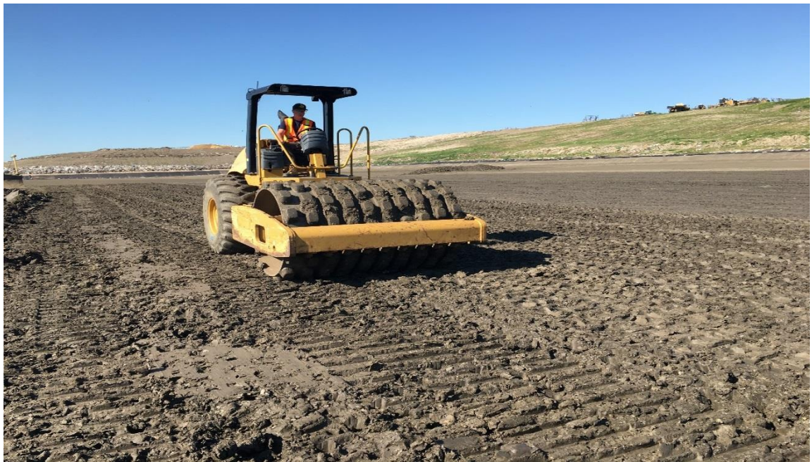
Compaction of Cell floor
