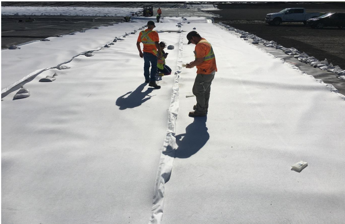
Installation of Geocomposite
