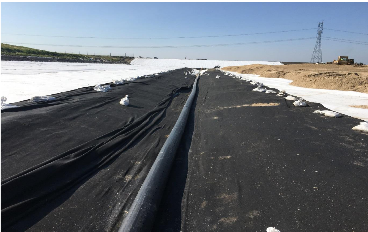
Leachate Collection Trench pipe and Geocomposite
