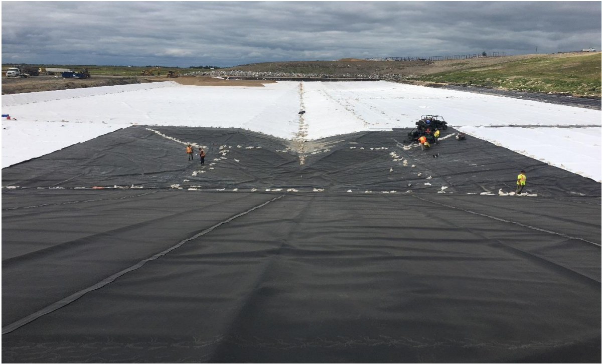
Completed Sump and Geocomposite on Floor
