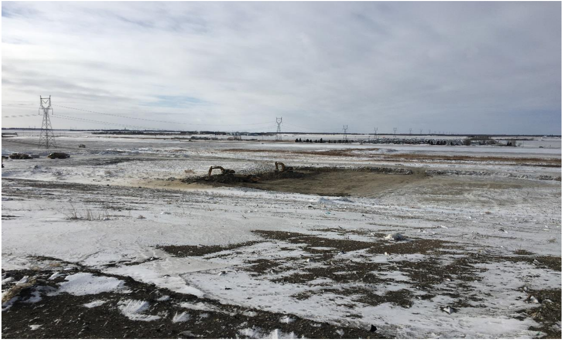
Winter Excavation of Cell 15
