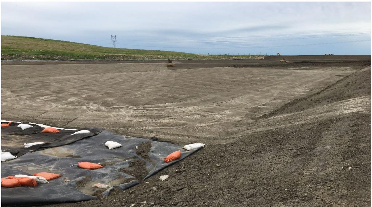
Preparing Cell floor for GCL deployment
