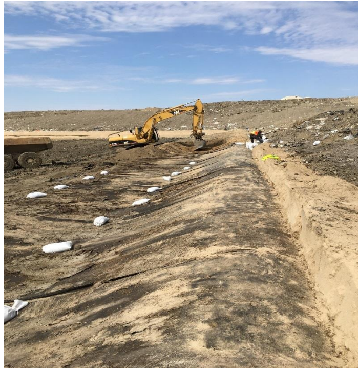
Removing sand from east tie-in to Cell 13
