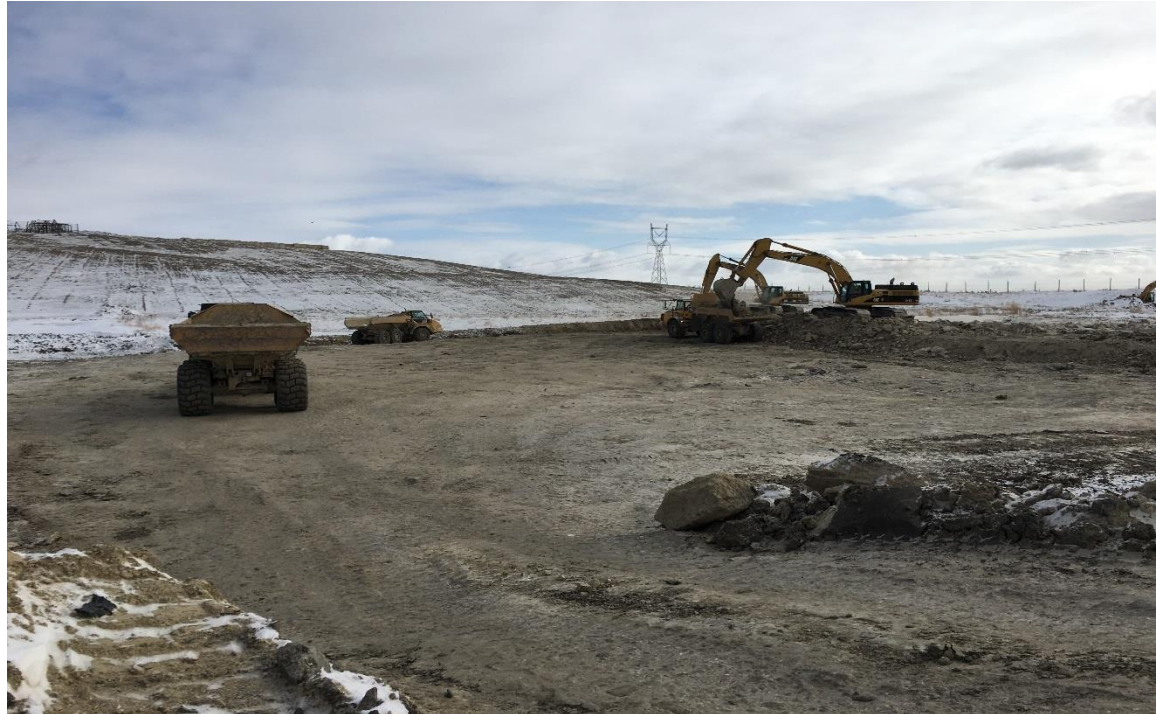
Winter Excavation of Cell 15
