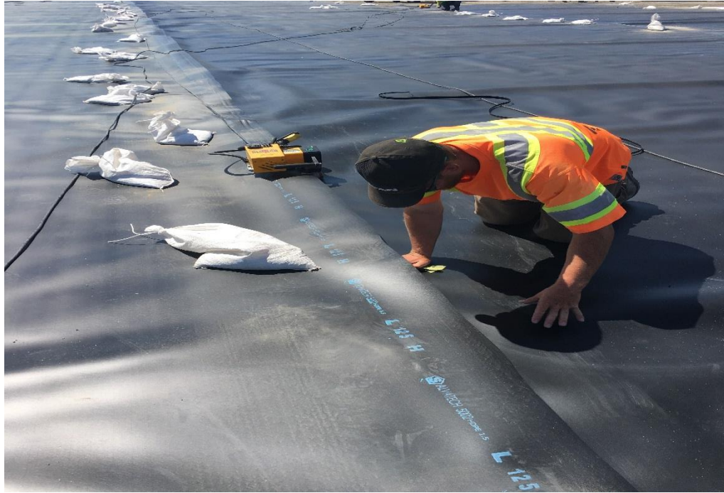
Fusion welding of seam
