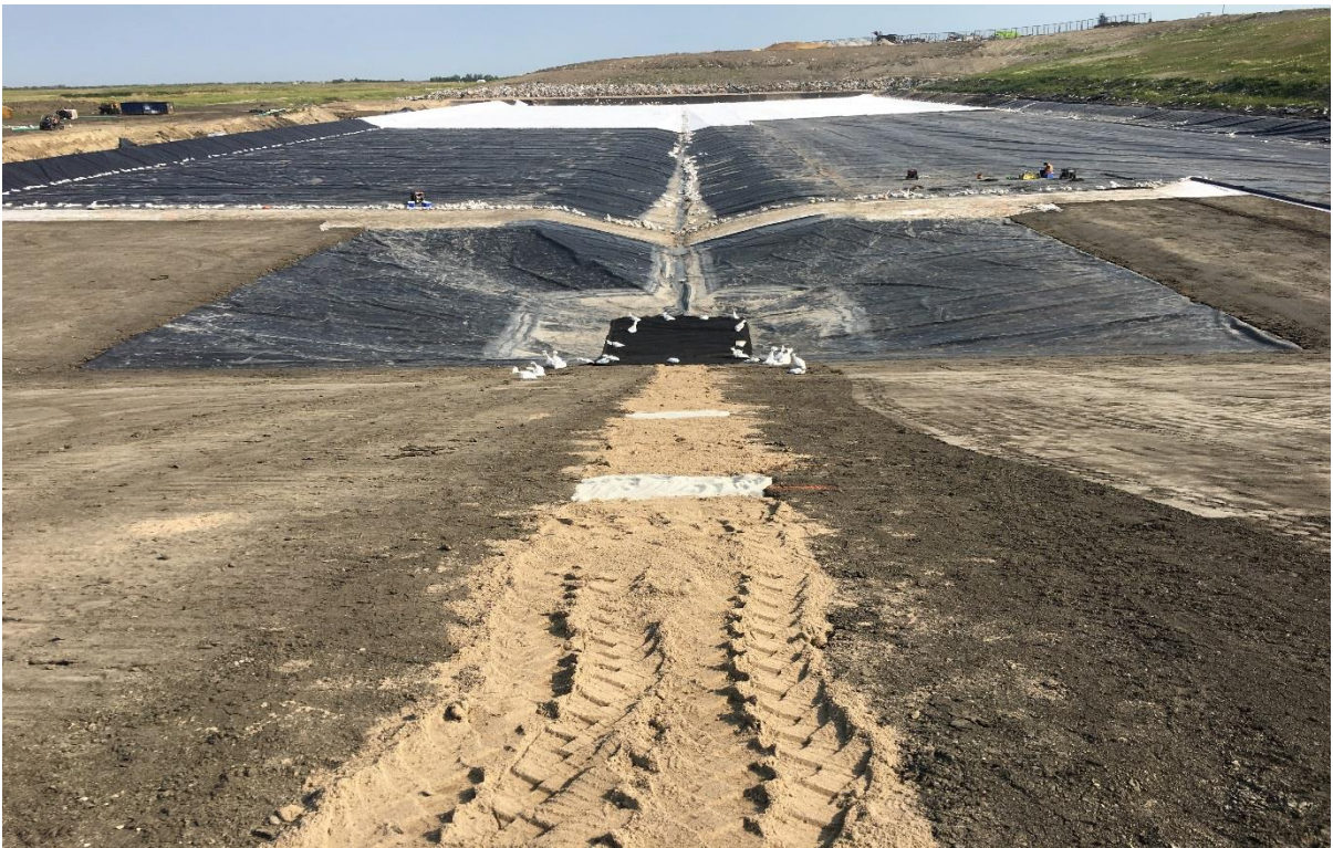
Completed Sub-liner Pipe installation
