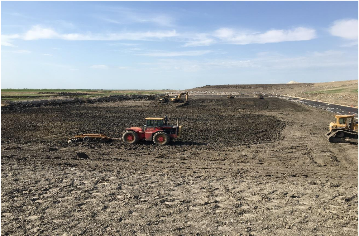
Excavation and conditioning of the cell floor looking North.
