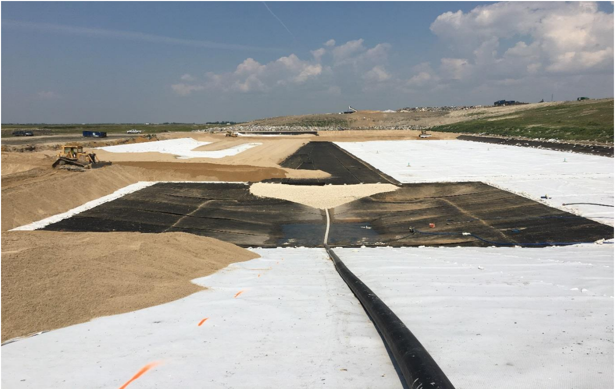
Sand Drainage layer installation
