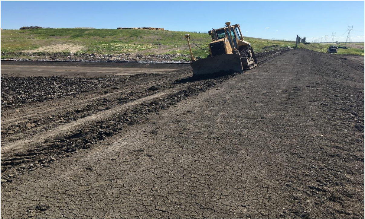
Trimming South Permanent Berm
