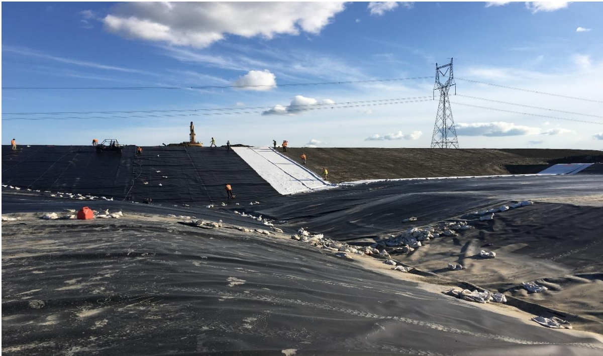
Deployment of GCL and HDPE geomembrane of South Permanent Berm
