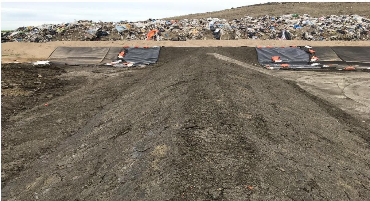
West Separation Berm tie into Cell 14
