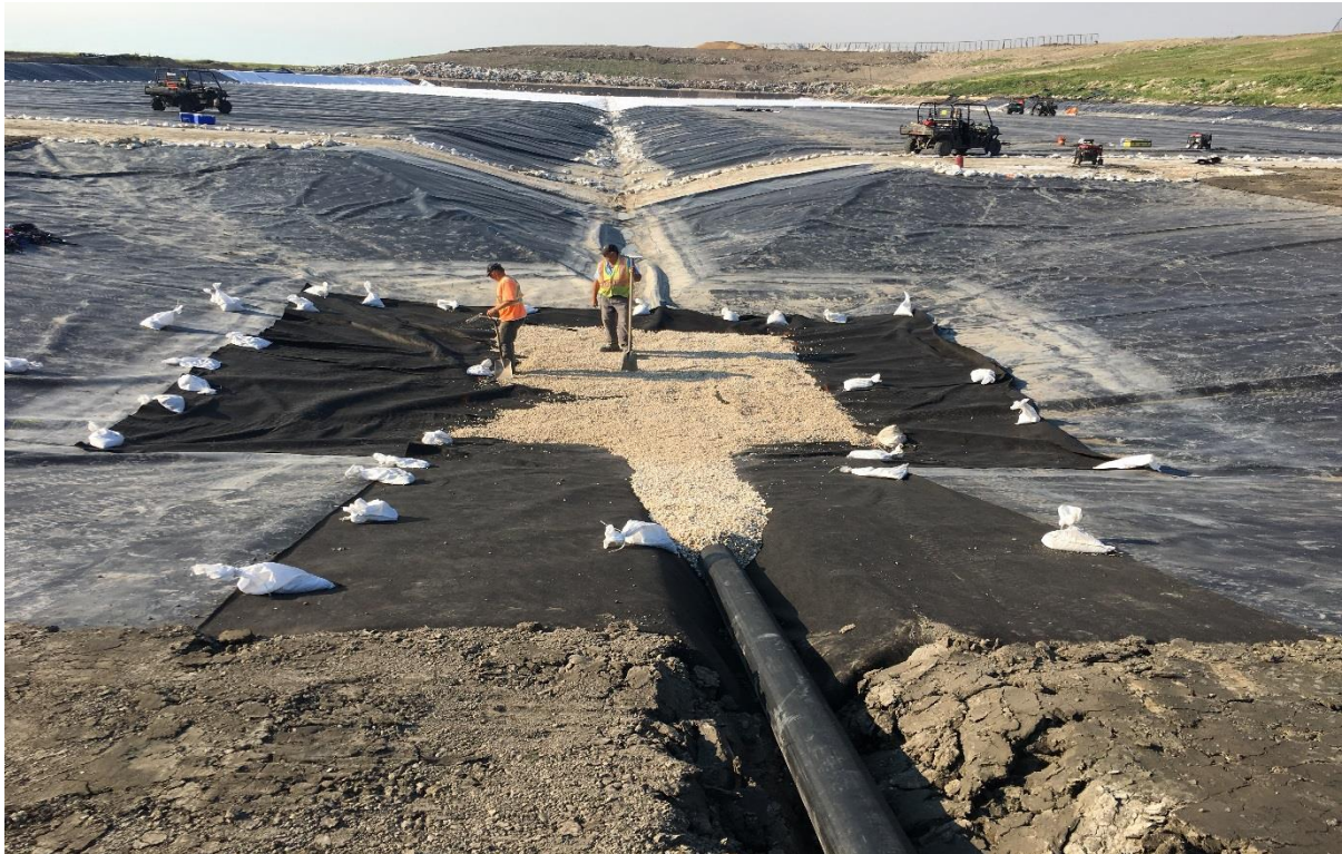
Placement of Sub-liner stone in Sump
