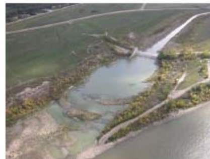
Floodway Channel Outlet shown during normal water levels. The outlet is located just downstream of the Lockport control structure on the Red River.
