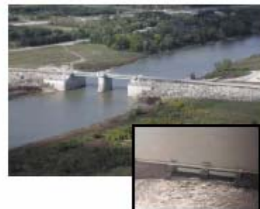
Floodway Gate Control Structure shown (top) under normal water levels, and (right) during 1997 Flood operations.
