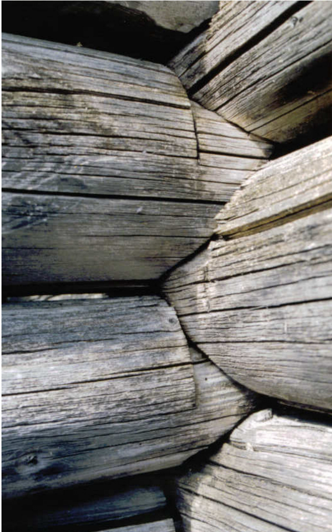
Plate 14: Detail of Log Construction
