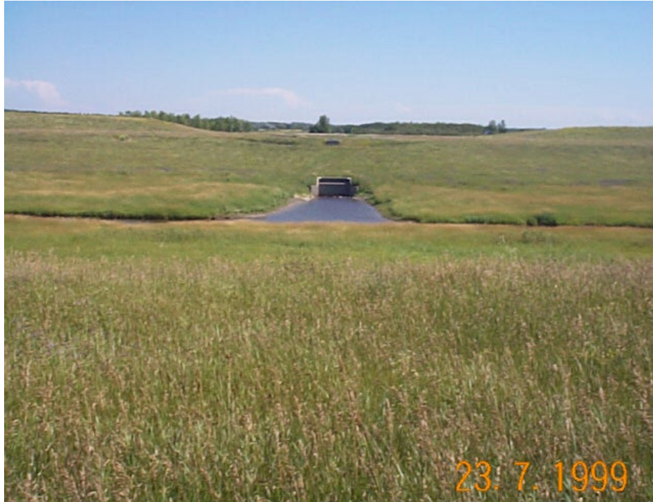
PHOTO NO. 7 TYPICAL DRAINAGE STRUCTURE ON EAST BANK OF FLOODWAY (LOW FLOW CHANNEL FLOWS FROM RIGHT TO LEFT)
