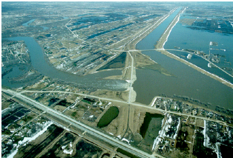
PHOTO NO. 8 FLOODWAY INLET IN 1997 FLOOD EVENT - INLET CONTROL STRUCTURE IN FOREGROUND - WINNIPEG TO LEFT (NORTH) - FLOODWAY FLOWS TOWARDS TOP OF PHOTO
