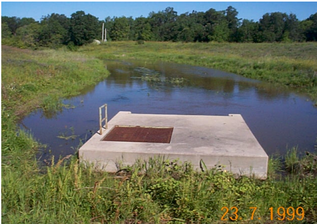
PHOTO NO. 2 SEINE RIVER INVERTED SIPHON OUTLET – RIPARIAN FLOW PASSES INTO SEINE RIVER IN BACKGROUND
