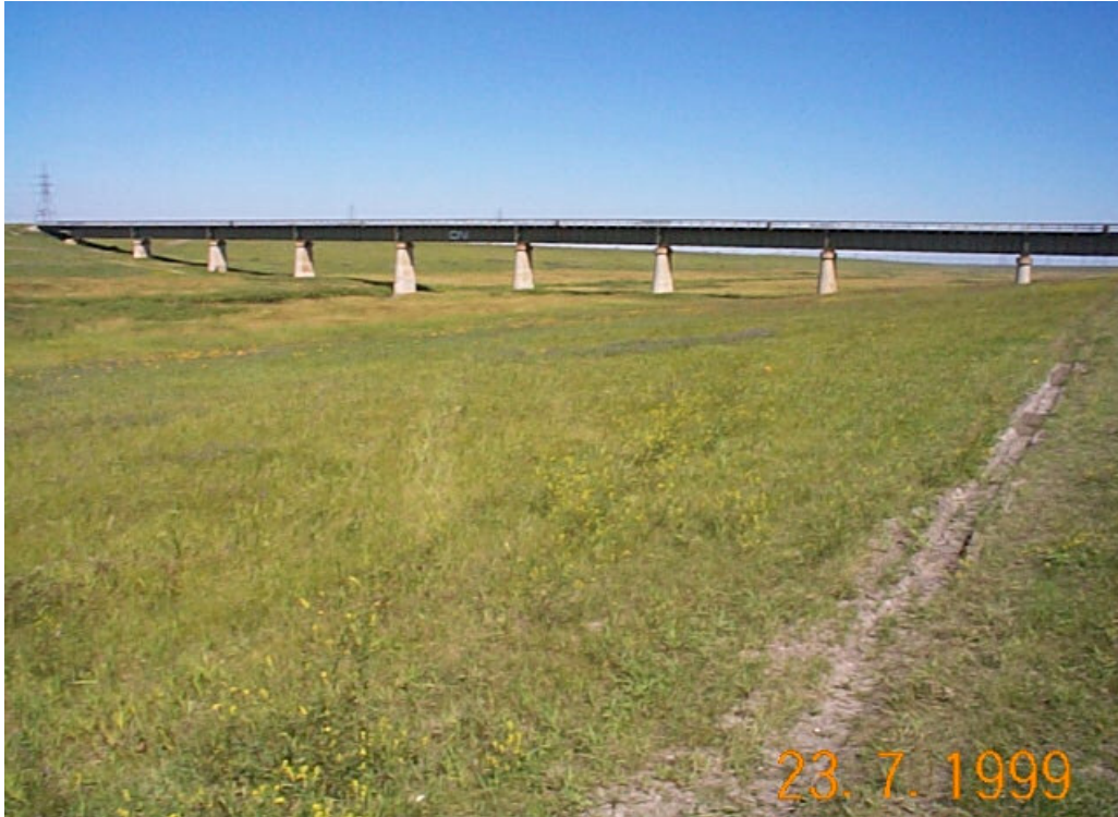
PHOTO NO. 9 TYPICAL RAILWAY BRIDGE OVER FLOODWAY
