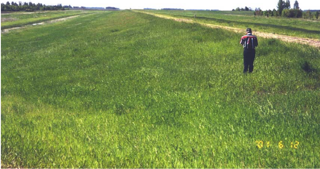
PHOTO NO. 5 WEST DIKE – SHOWS TYPICAL HEIGHT AND SIDE SLOPES
