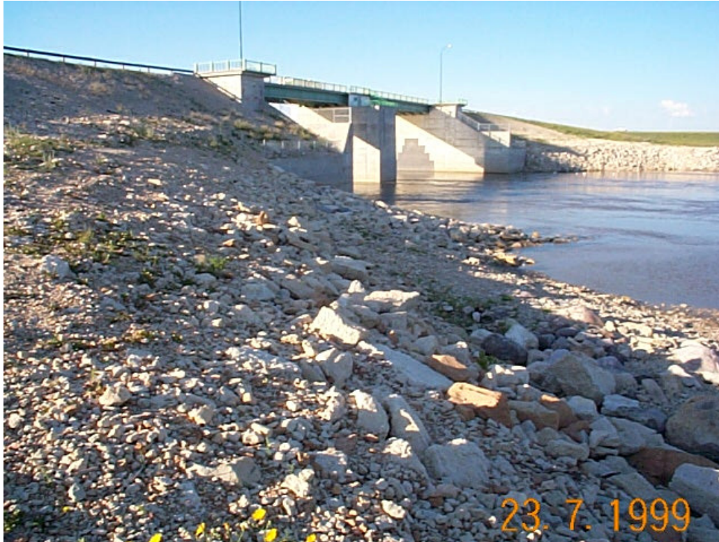
PHOTO NO. 1 FLOODWAY INLET CONTROL STRUCTURE (DOWNSTREAM SIDE)
