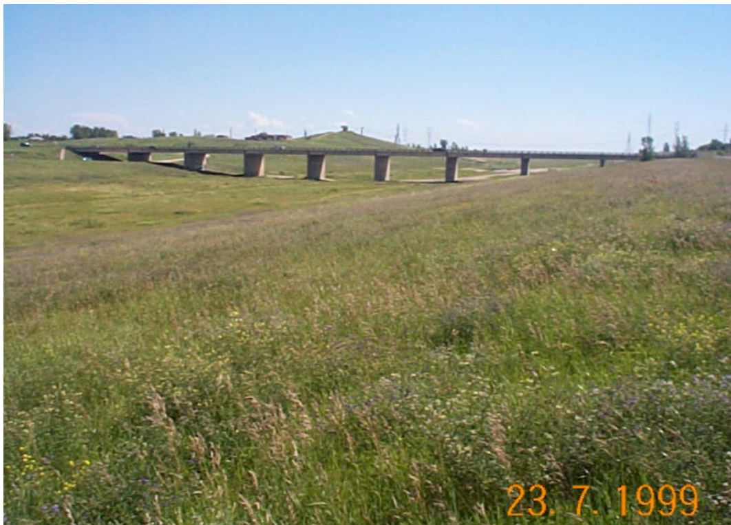
PHOTO NO. 6 FLOODWAY AT PTH 59 NORTH; SKI HILL IN BACKGROUND
