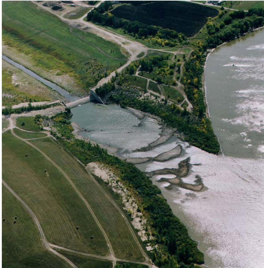
PHOTO NO. 4 FLOODWAY OUTLET STRUCTURE
