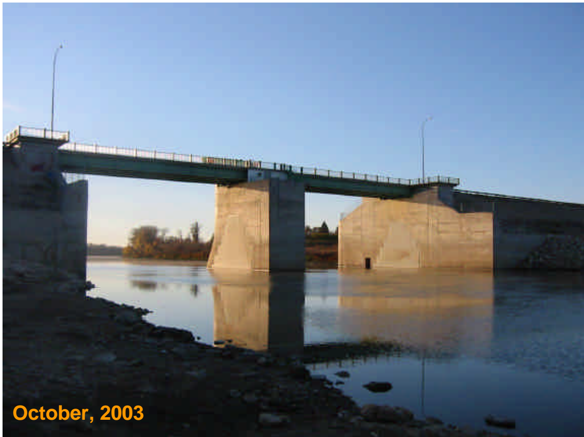
Red River Floodway Inlet Control Structure Inactive Operations Figure 1-3
