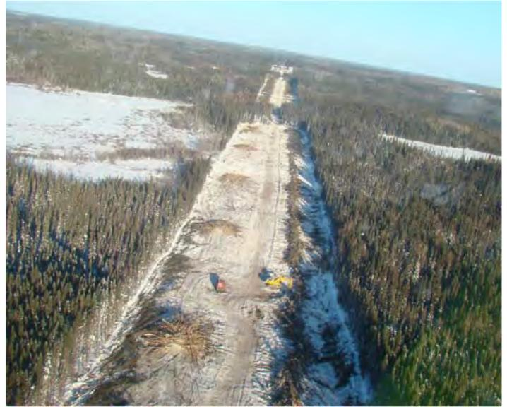
**Photo 4: Aerial Shot of Clearing of Bipole III Transmission Line**
