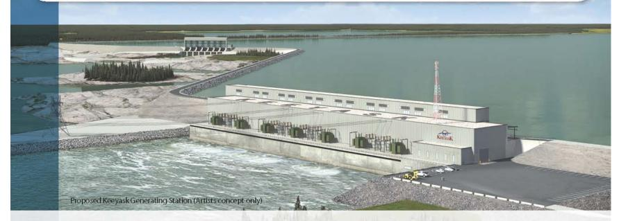
The Keeyask Hydropower Limited Partnership is proposing to develop the Keeyask Generation Project, a 695-megawatt hydroelectric generating station at Gull Rapids on the Nelson River in northern Manitoba.
