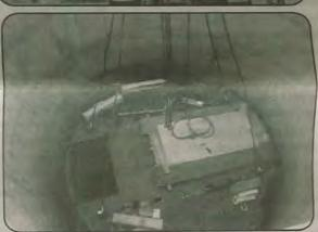
(L): Lalor Project Manager, Kim Proctor ~ photo by Marc Jackson (Top R): Placing Top Deck on Galloway - April 10, 2011 (Bottom R): Galloway in Shaft - April 10, 2011 ~ HudBay Minerals photos (ED NOTE: Galloways are used as temporary working platforms in vertical shaft development. As vertical development progresses, the Galloway is lowered as required.)
