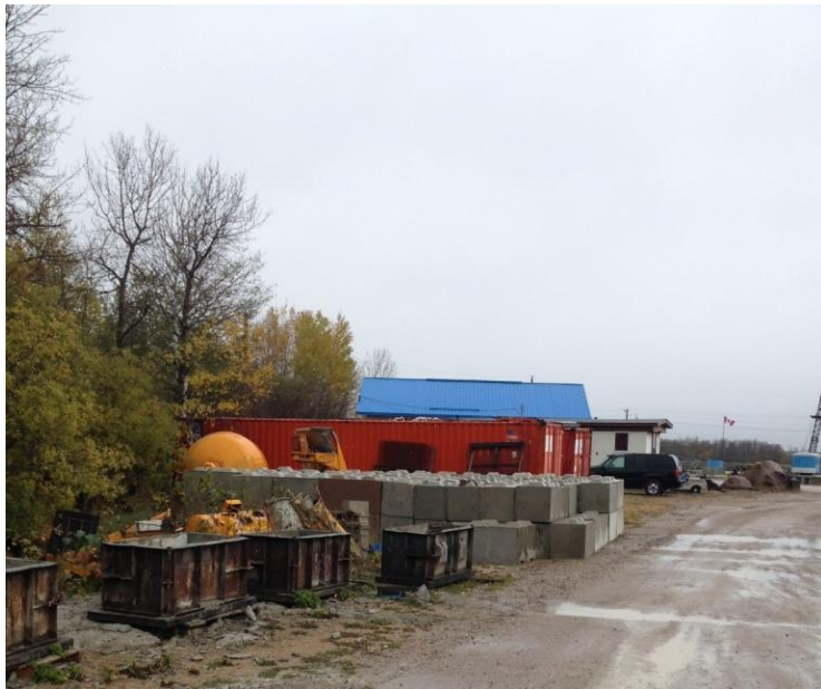
Excess concrete used for concrete blocks
