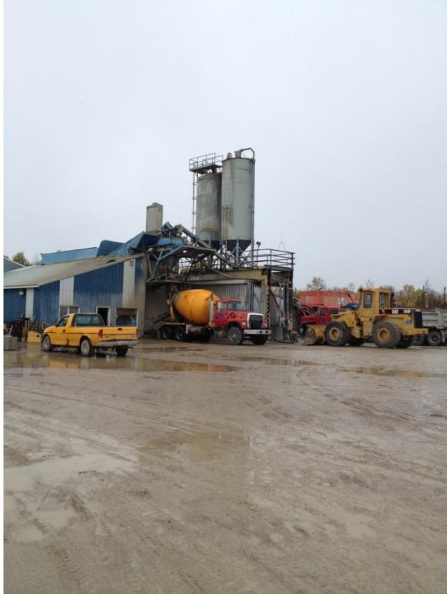
View of plant from south
