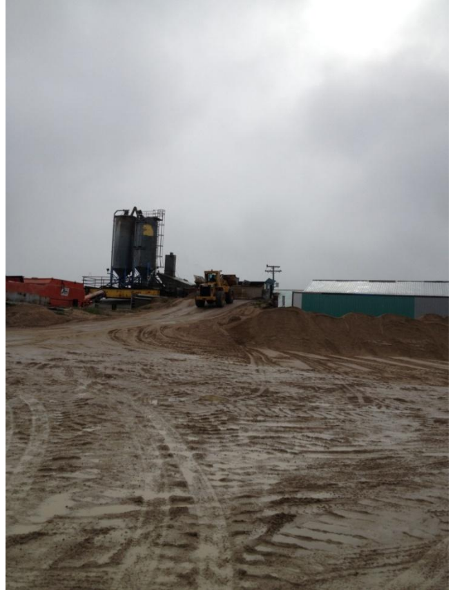
View of plant from north
