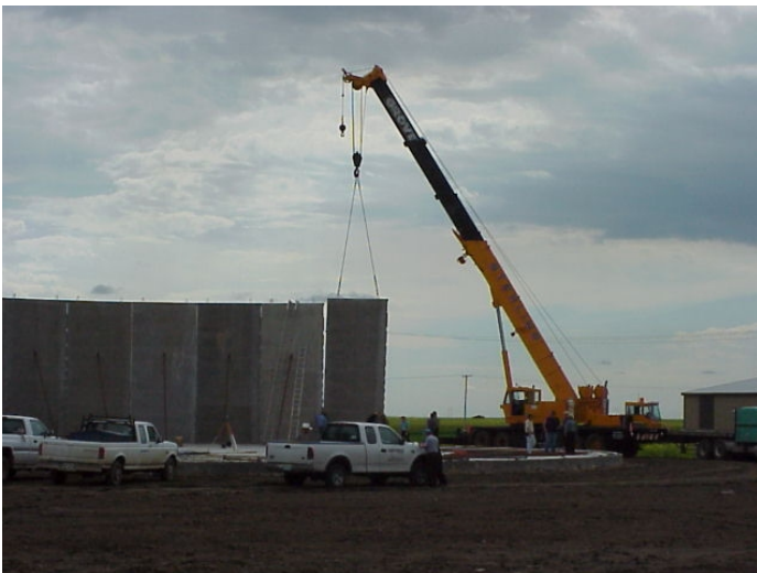
Pre-cast panels for circular concrete storage structures
