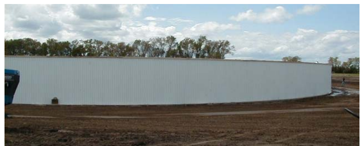
Concrete storage structure with permanent plastic forms
