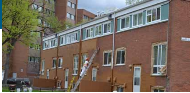
Construction worker upgrading exterior of units at Lord Selkirk Park
