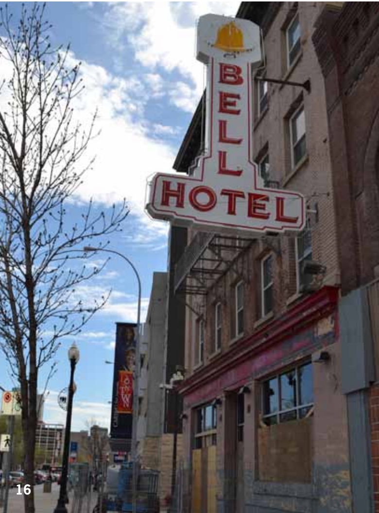
Bell Hotel undergoing renovations funded by Manitoba Housing
