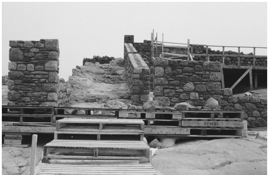
Figure GS-39-6: Brian Ladoon's hotel site, front entrance.
