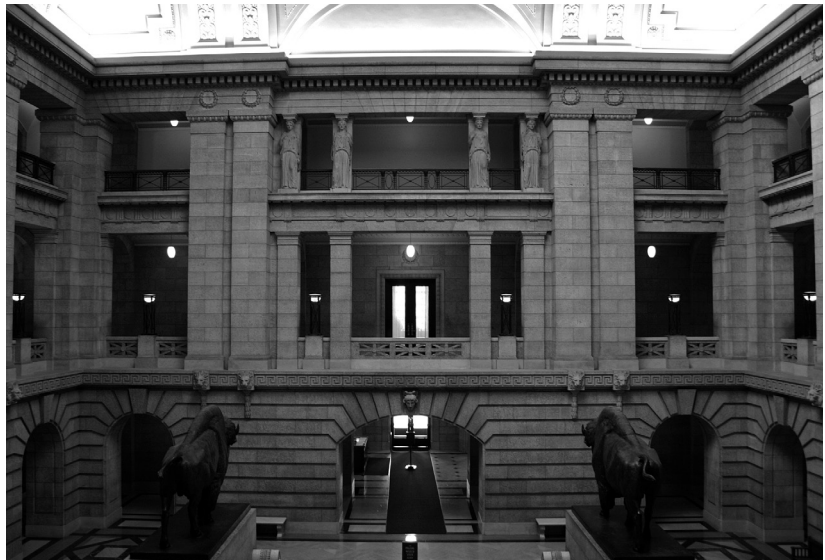
Figure 15: View from the top of the Grand Staircase. Tyndall Stone is the dominant dimension stone used in the Legislative building. It is used on walls, arches, columns, gallery balustrades and sculptured forms. The floors at the bottom of the staircase are Tennessee marble, Ordovician black marble and green Verde Antique marble. The four caryatids on the top floor are carved from Bedford limestone. Field trip Stop 2.
