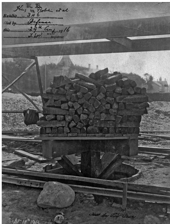
Figure 6: Loaded platform for the bearing test on indurated till in the excavation for caisson 39, located adjacent the north portico along the northeast wing (Archives of Manitoba, GR3085 G8101, Item 28). The test was done using a progressively loaded platform, 1.68 m square, that was erected on a 3 x 3.6 m rectangular mast extending to indurated till (Archives of Manitoba, GR3085 G8100, Item 6). An initial 5 tons of pig iron was placed on the mast and 22 mm of settlement occurred after 3.5 hours. Another 10 tons of pig iron were added at intervals over the next 24 hours. A total of 26 mm of settlement was measured during the 44 hours of the test. Upon removal of the load 6 mm of rebound was measured. Wood cribbing and metal rings support the wall of the caisson excavation.
