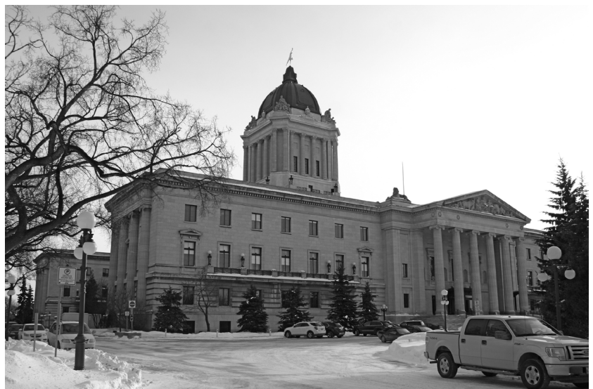
Figure 11: The Manitoba Legislative Building, viewed from the site of the northwest corner of the second Manitoba Parliament buildings, winter 2013. Field trip Stop 1.
