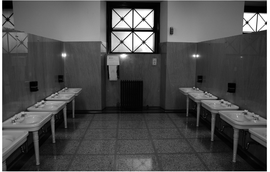
Figure 30: Walls in the public washrooms are lined with red Tennessee marble. The marble displays many of the common features of the pink Tennessee marble that occurs in the Rotunda. Terrazzo forms the square floor tiles. Field trip stop 10.
