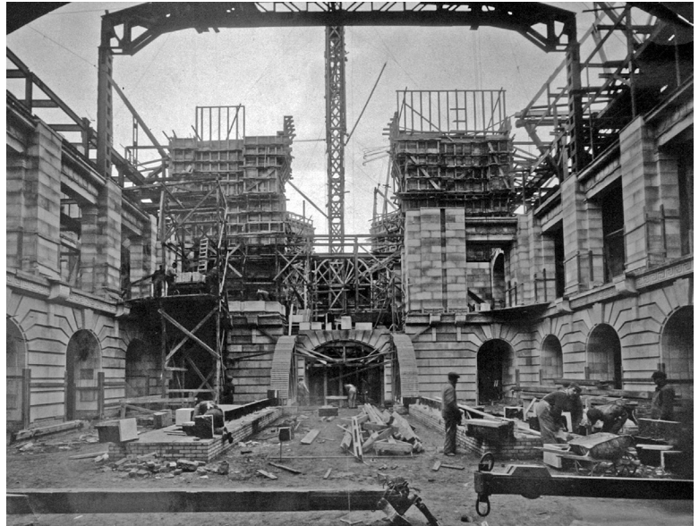
Figure 3: 1916; the Grand Staircase area on the main floor. (Archives of Manitoba, Foote Collection 78). Workers lay brick and steel supports to prepare the base of the Grand Staircase for its railings, addition of the Tyndall Stone facing and placement of the two bronze bison that flank the staircase (see Figure 8a).
