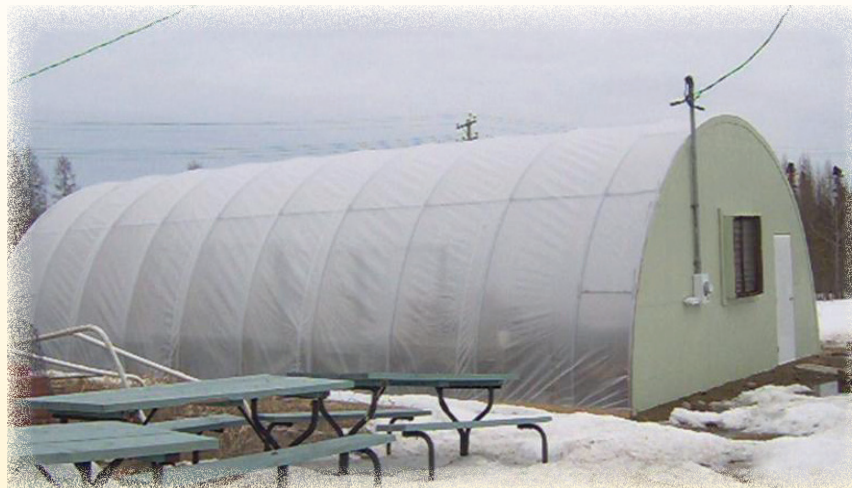
Refurbished greenhouse in Wabowden, MB
