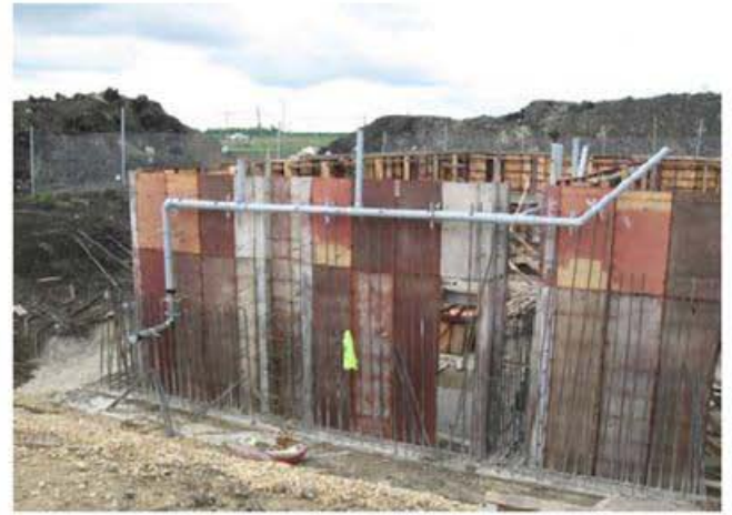
St. Clements Water Treatment Plant
