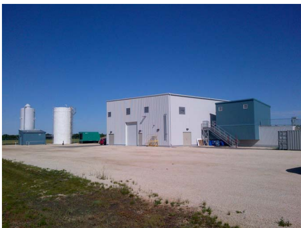
Headingley Wastewater Treatment Plant
