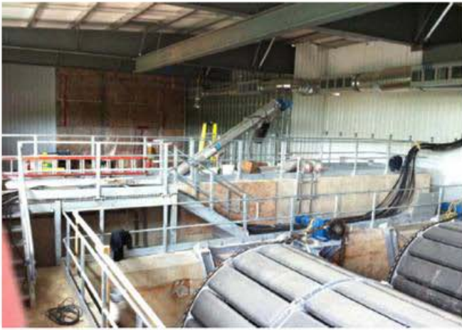
Snow Lake Wastewater Treatment Bio-wheels
