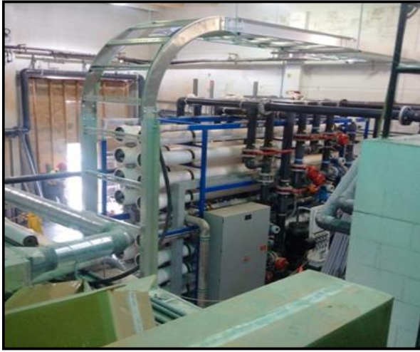
South Central District Water Co-op Water Treatment Plant Upgrades
