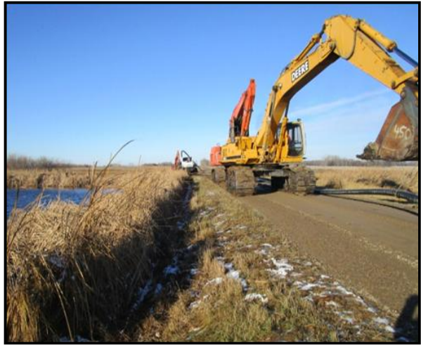
Whitehead Rural Water Pipeline
