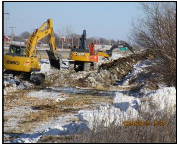
Pipestone Rural Water Pipeline
