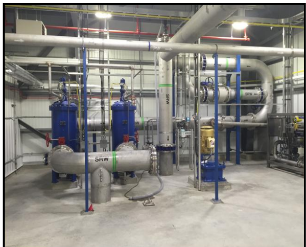
Cartier Regional Water Expansion Headingley Water Treatment Plant
