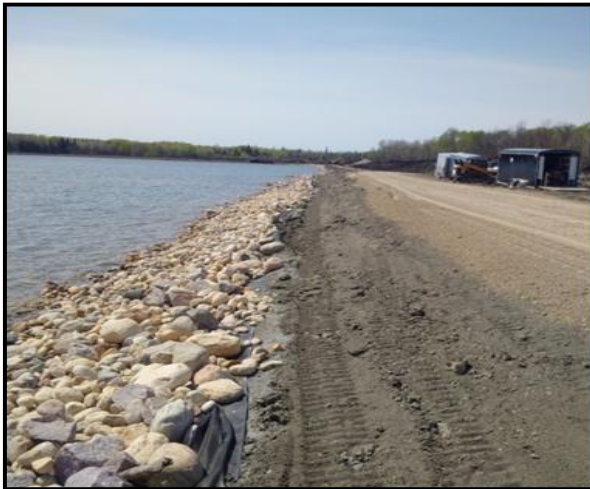
Pinawa Wastewater Lagoon Upgrade
