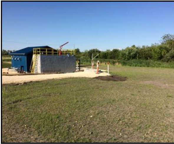
Winnipeg Beach Wastewater Lagoon Upgrades
