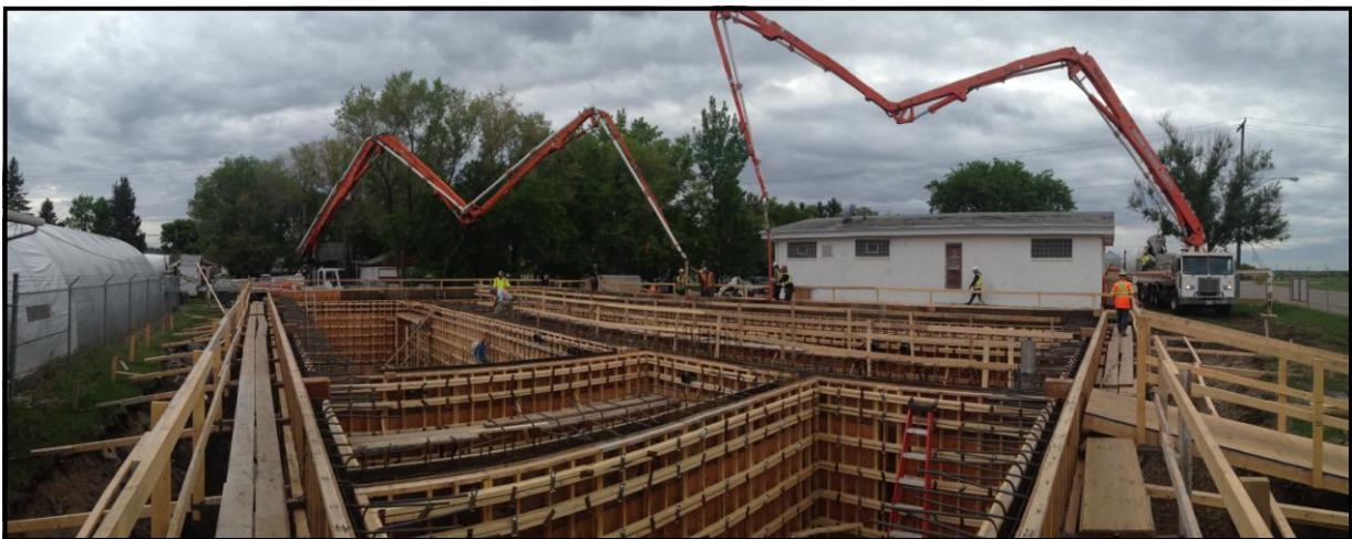
Rivers Water Treatment Plant
