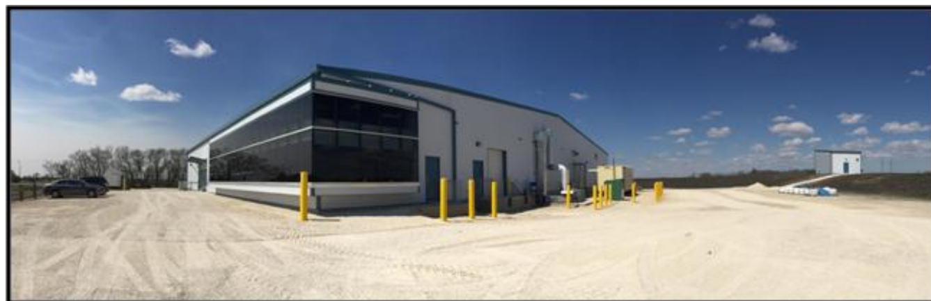
Cartier Regional Water Co-op Headingley Water Treatment Plant
