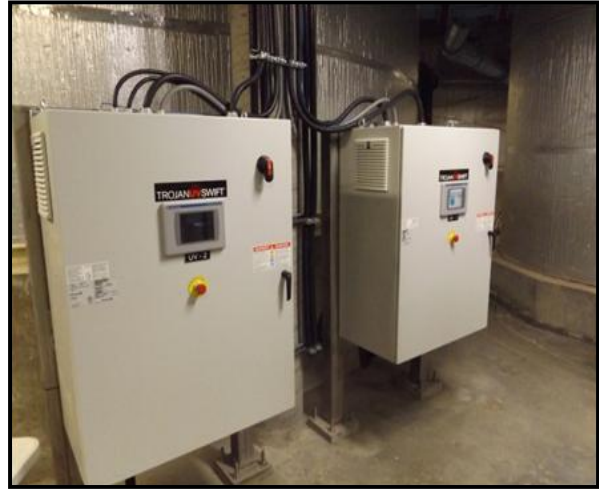
Morden Water & Wastewater System Upgrades - UV Treatment
