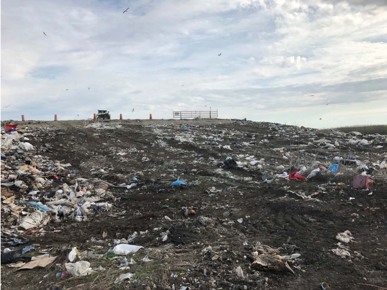
Temporary Cover on Active Face
