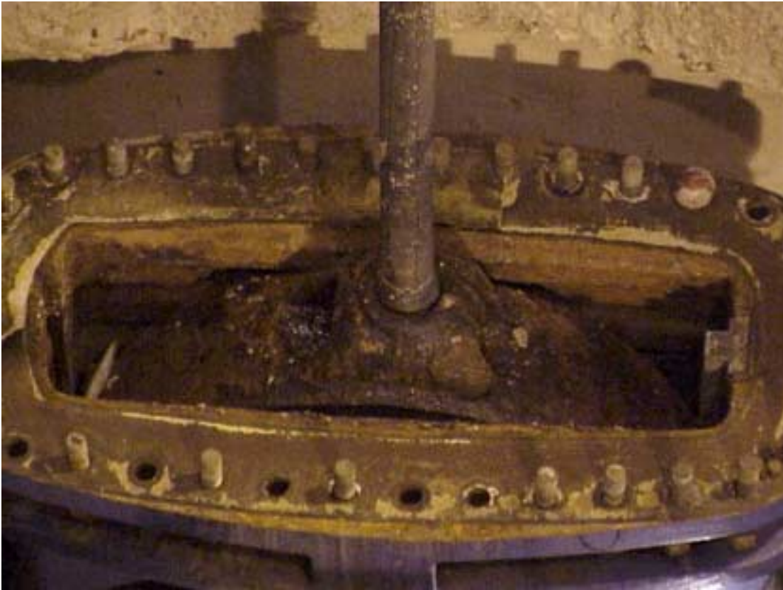
Viewing into the lower portion of suction gate valve.
