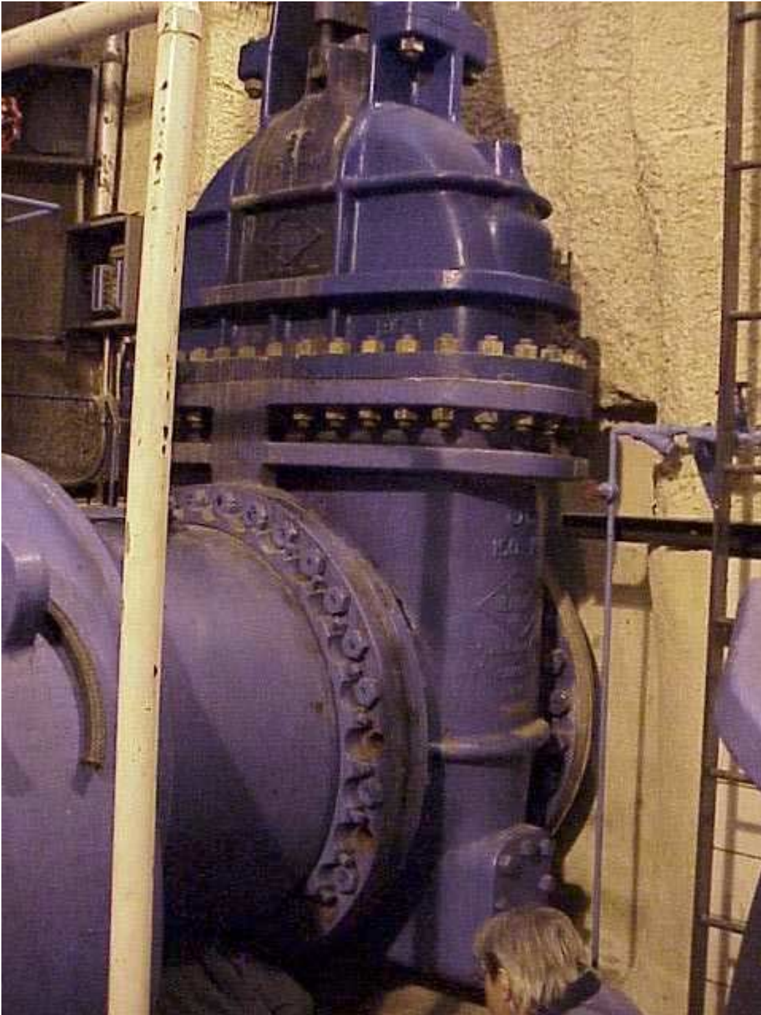
Suction gate valve and reducer - white pipe is designed to drain wastewater located between the discharge side of the suction gate valve and the discharge header.
