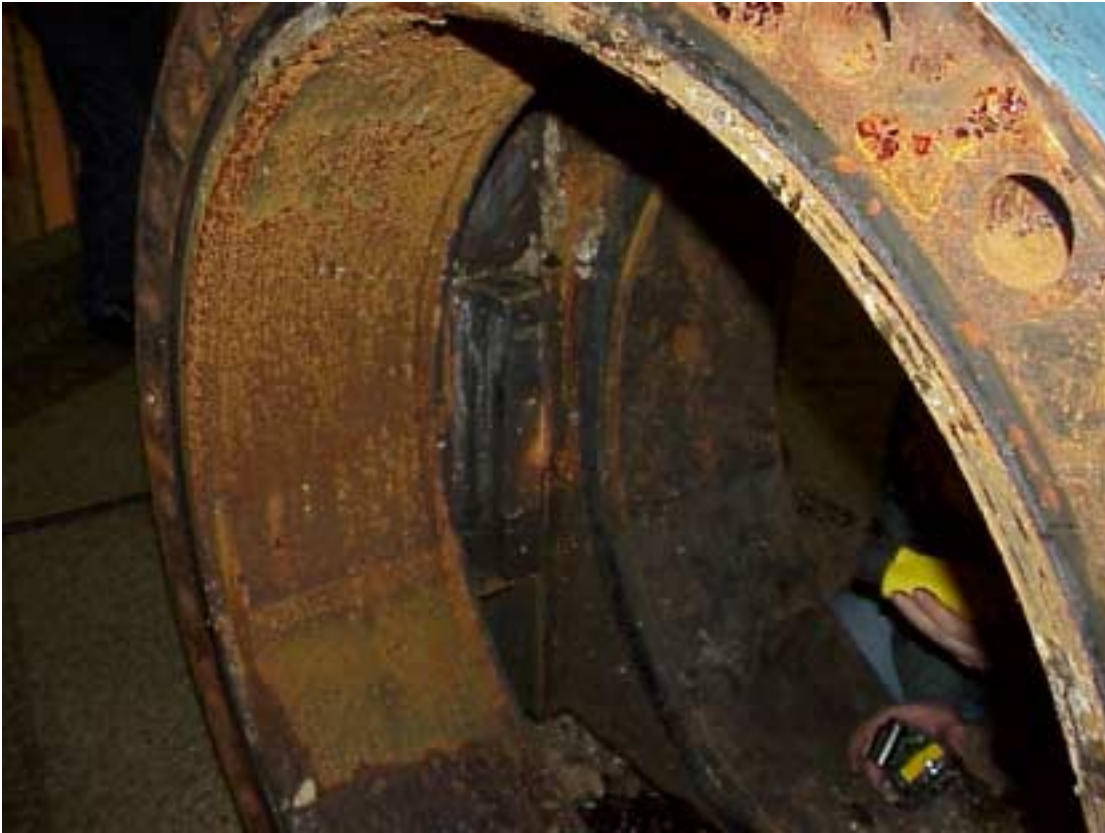
Valve body showing upper valve guide from bonnet now located in lower portion of valve body.
