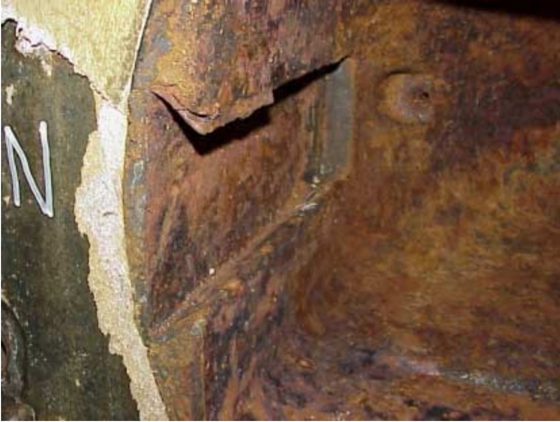
Close up view of valve bonnet showing channel where guide bar would be located.
