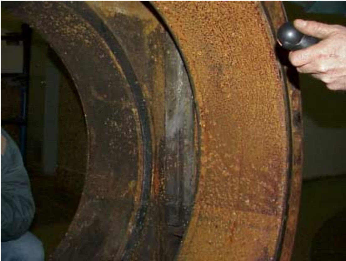
Valve guide bar in place on opposite side of valve body of suction gate valve.
