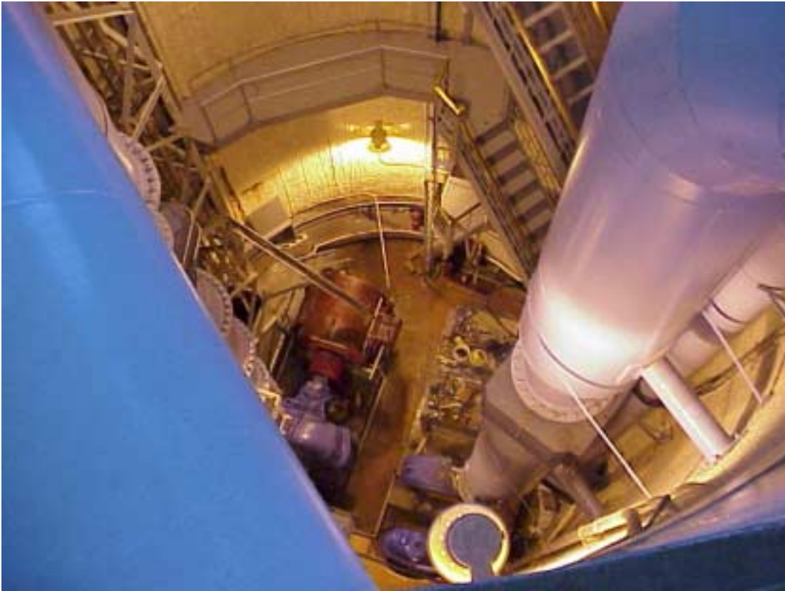
Viewing down into dry well, shows valve, reducer, pump attached to white discharge header on right side of photo.
