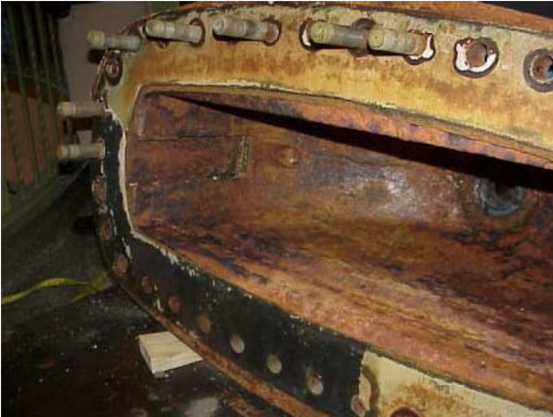
Interior view of valve bonnet showing location of where valve guide bar is missing from.
