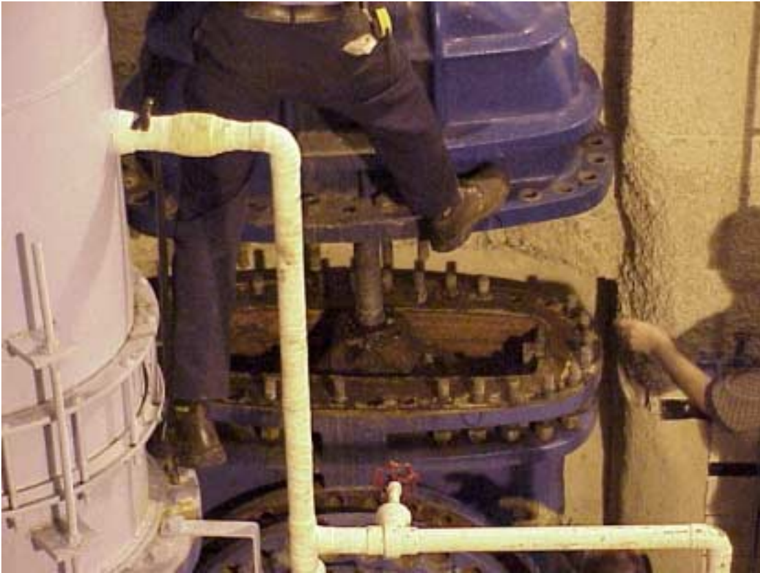
Removal of the valve bonnet - photo shows location of valve plate and attached valve stem.
