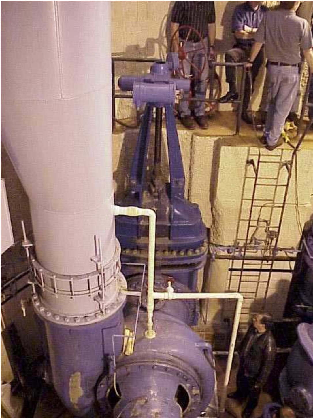
Photo shows suction gate valve in back and pump MP5 in foreground. Small diameter white pipe is the system drainage piping. The large white pipe on the left side of the photo is the discharge header. Inspection plate is located on the left side of the pump below the discharge header.
