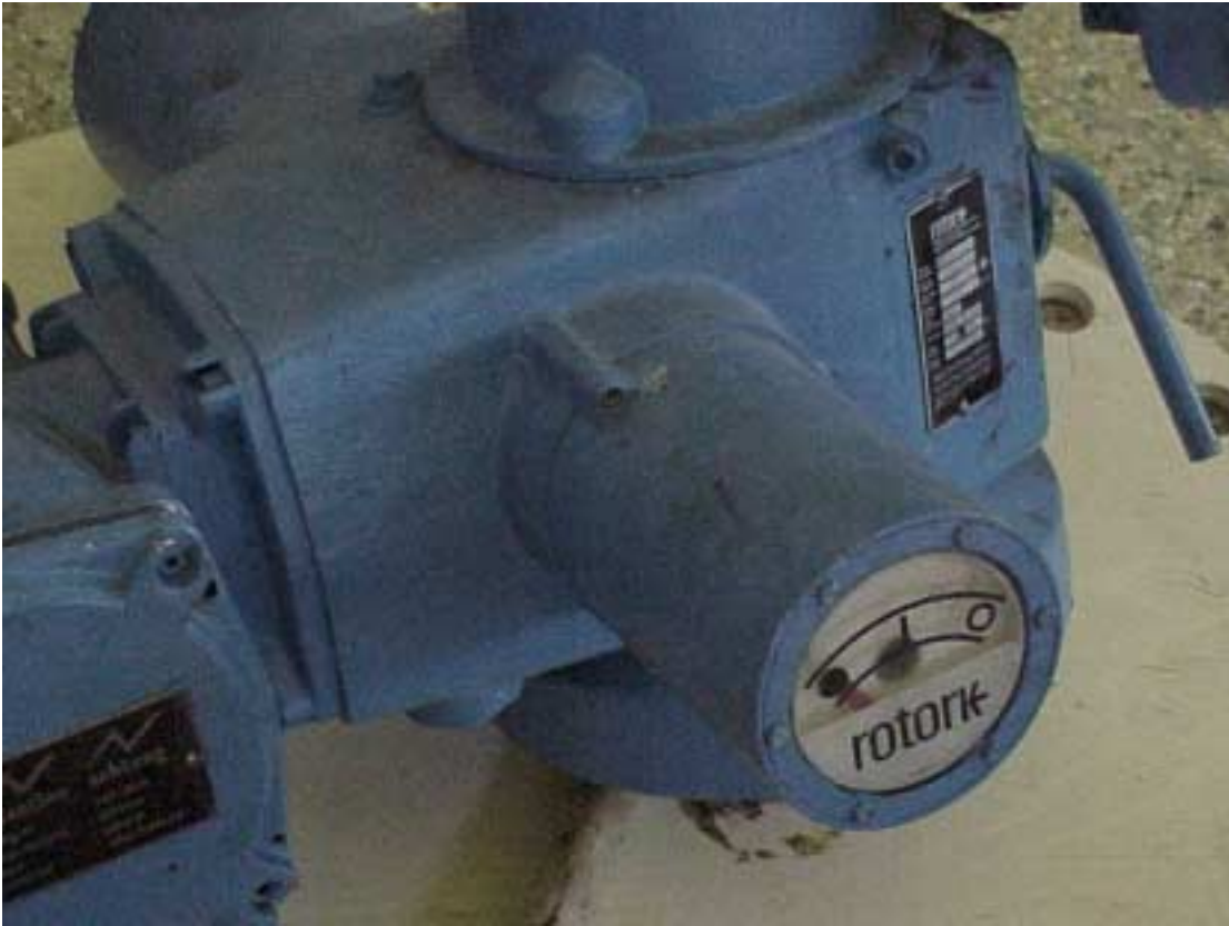
Rotork Actuator and valve position gauge.
