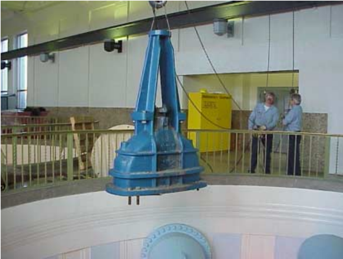
Valve bonnet being removed from dry well.
