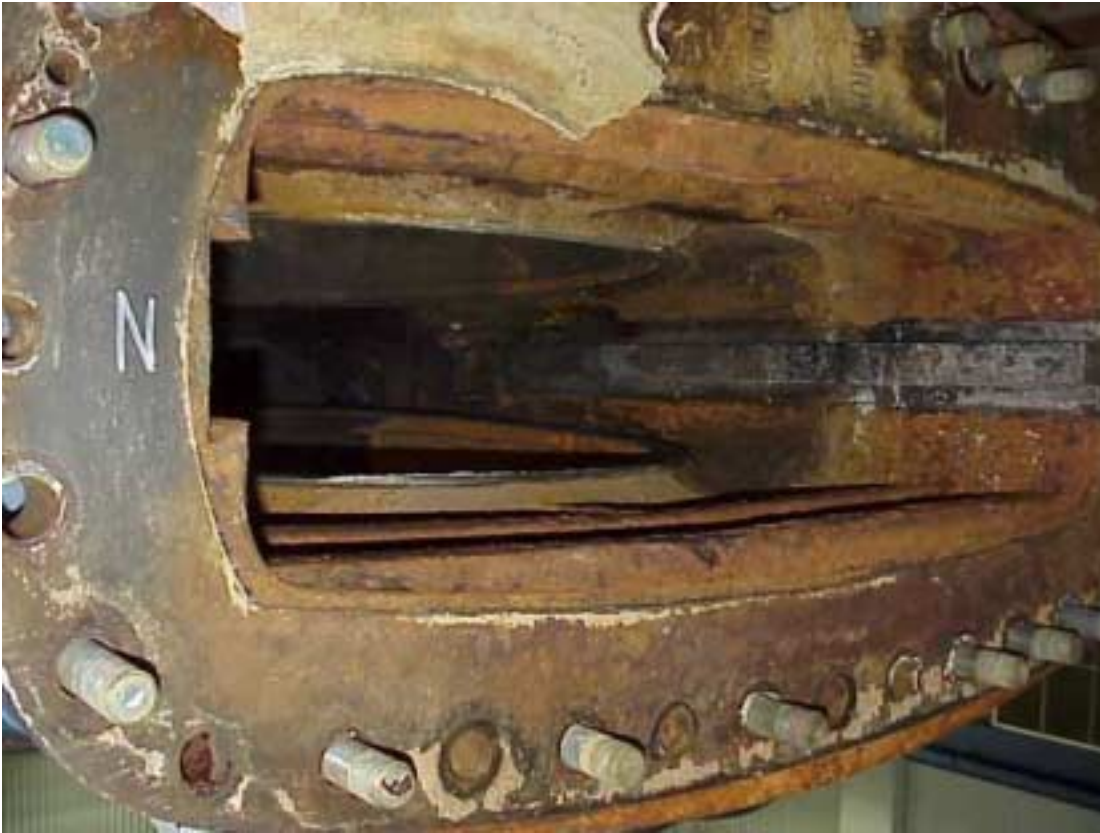
Lower portion of suction gate valve showing valve guide bar in place on right side of photo and missing on the left side of the photo. Guide bar would be located in the dovetail shaped channel.
