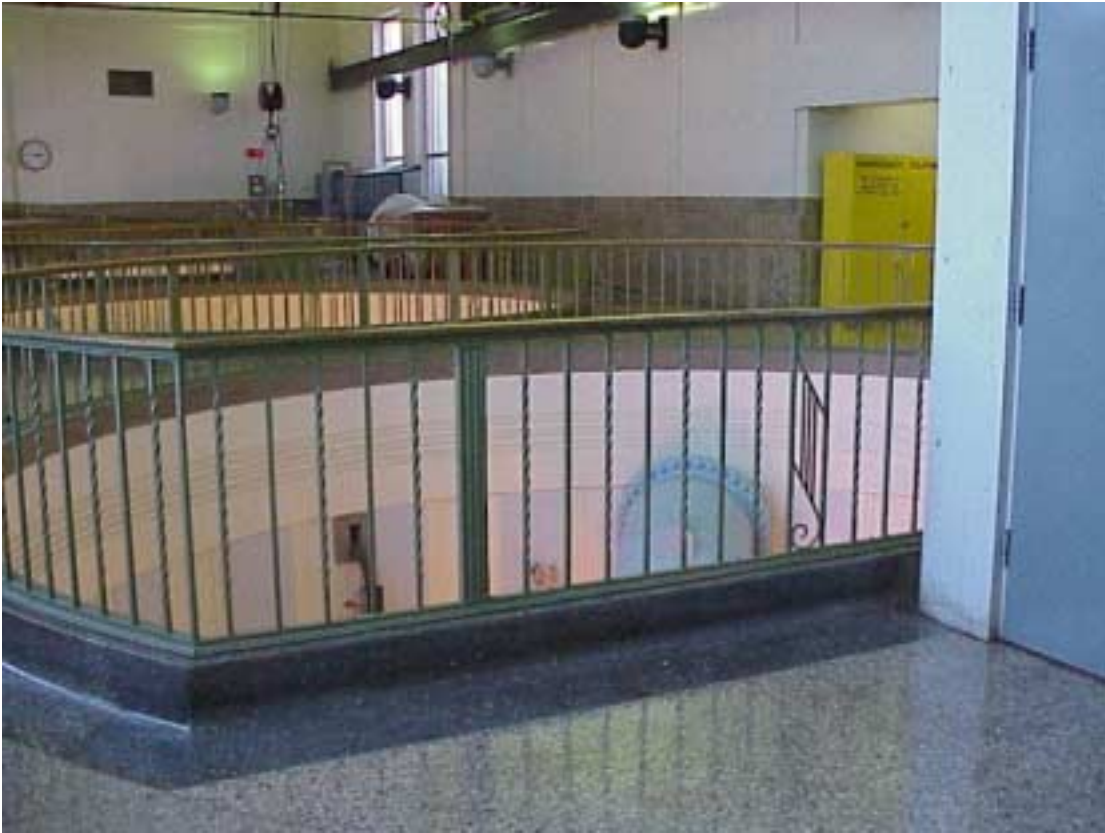
Three dry wells.
