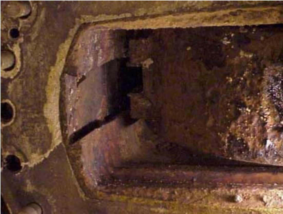
Photo shows valve guide missing from valve body.
