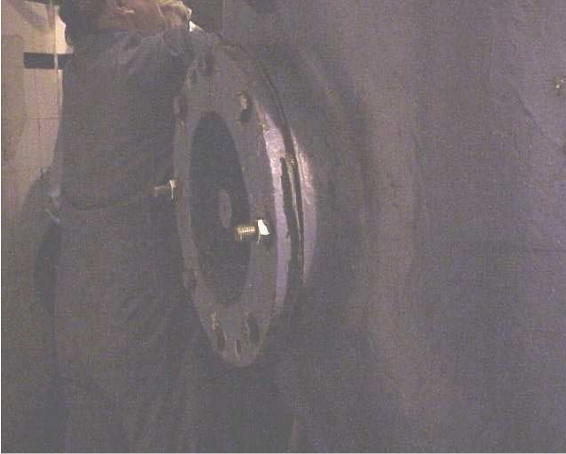
Inspection plate on the side of pump MP5.
