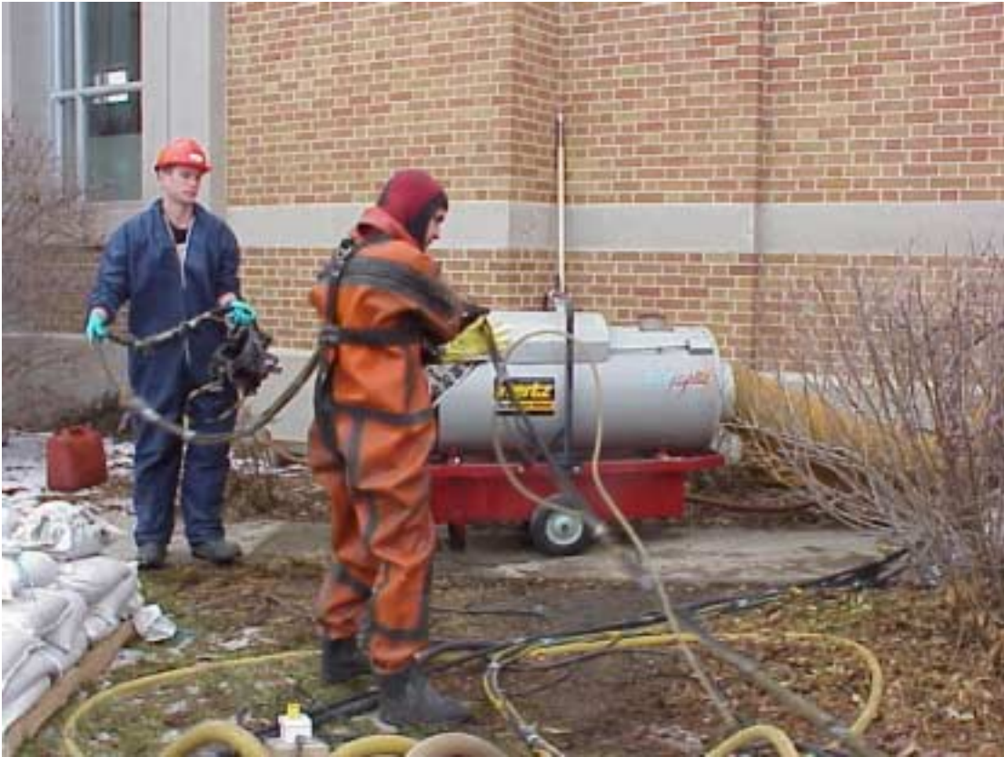
Commercial diver preparing to enter the east suction header.
