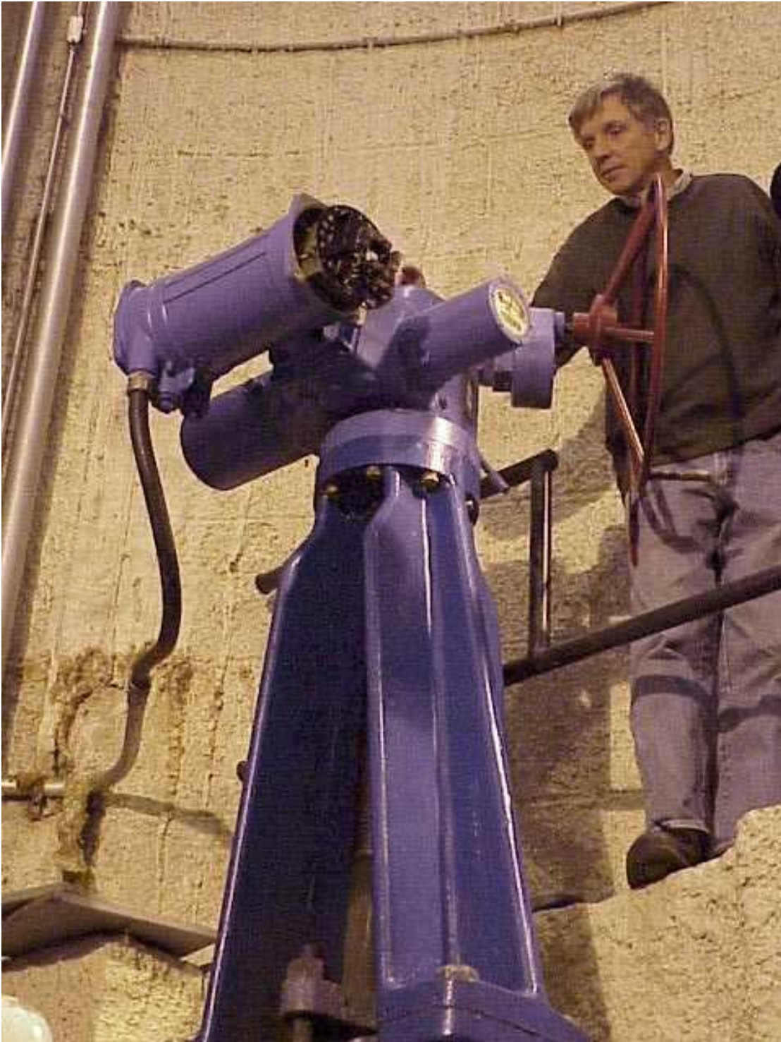
Rotork valve actuator and manual wheel located on top of valve stem guide assembly.
