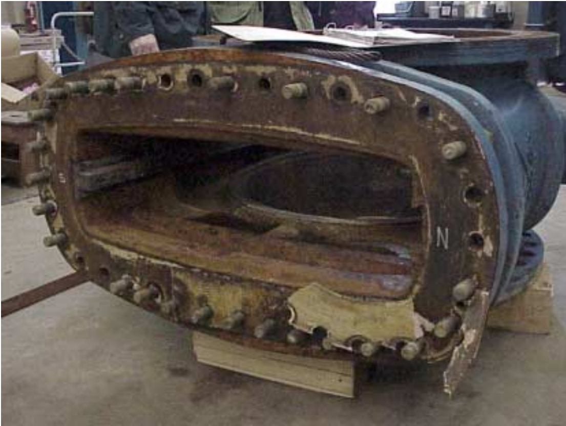
Photo of lower portion of suction gate valve body.
