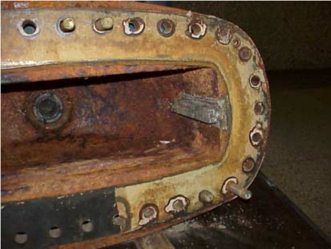
Opposite side of valve bonnet with valve guide bar in place.
