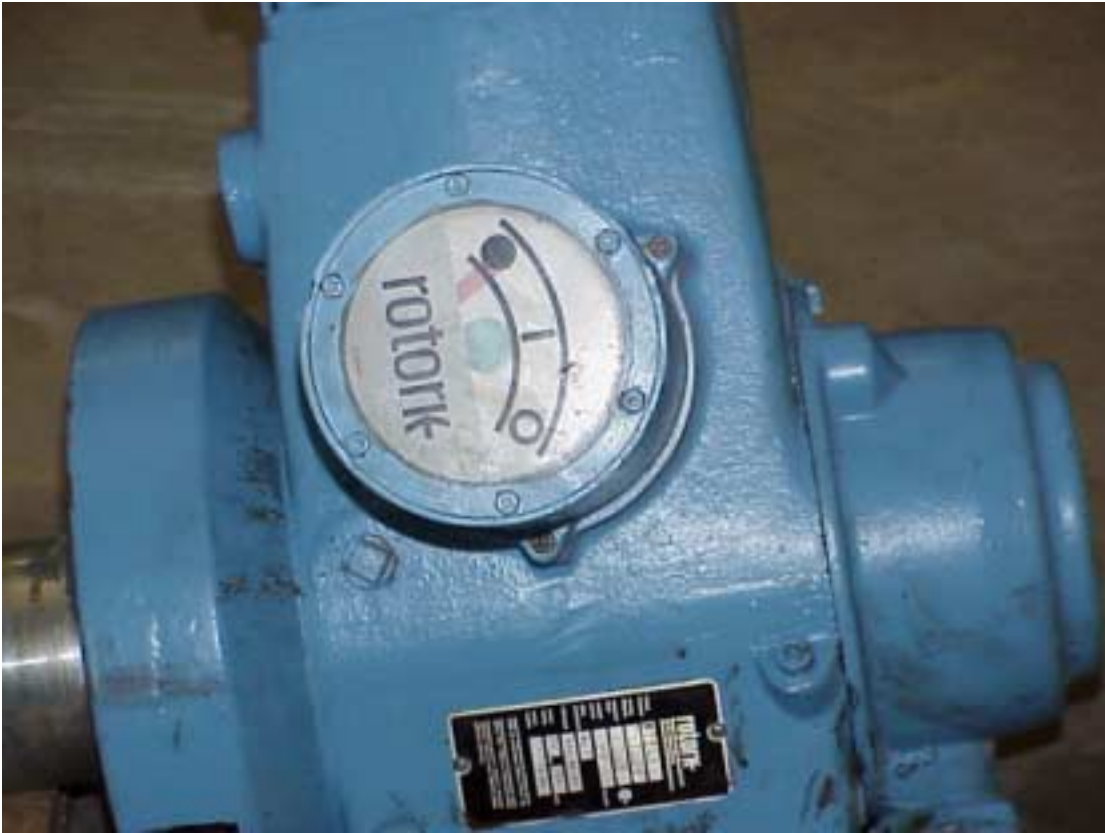
Close up view of valve position gauge on Rotork.
