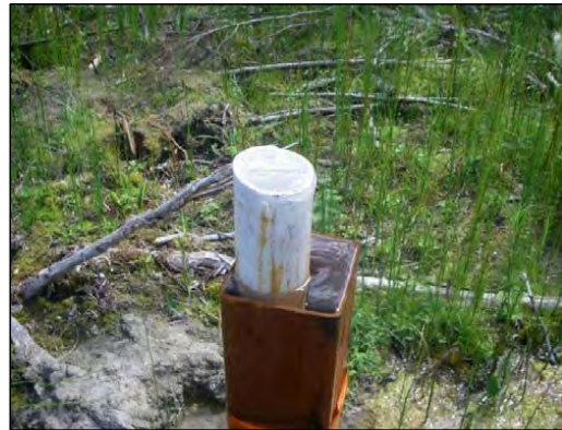
D. Flowing artesian conditions at MW-7-LS.
