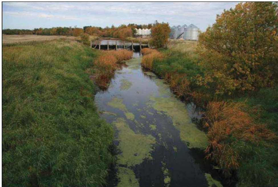
Figure 5-4: Stop-log dam on the La Salle River south of Elie.
