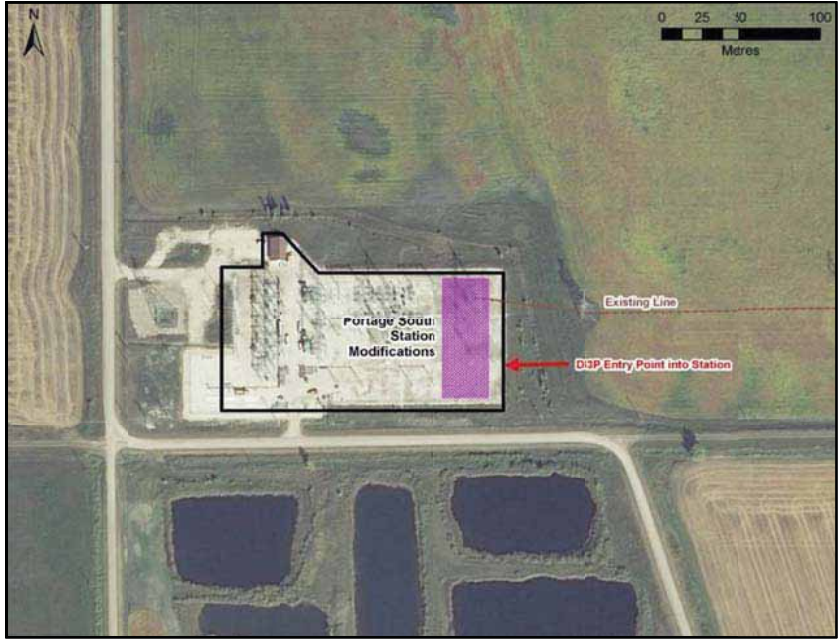
Figure 3-5 Locations of equipment additions and modifications to the Portage South Station.
