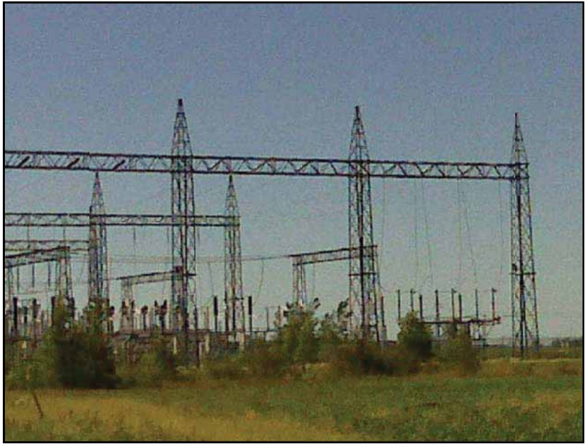
Figure 3-6 Ground view of the D83P ingress location to the Portage South Station.
