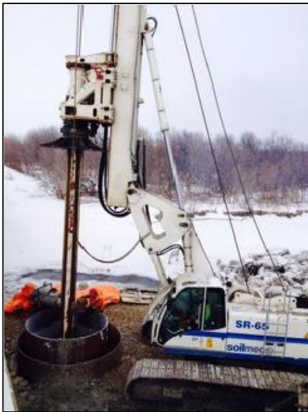
Photo 1: Example of drill unit to be used
