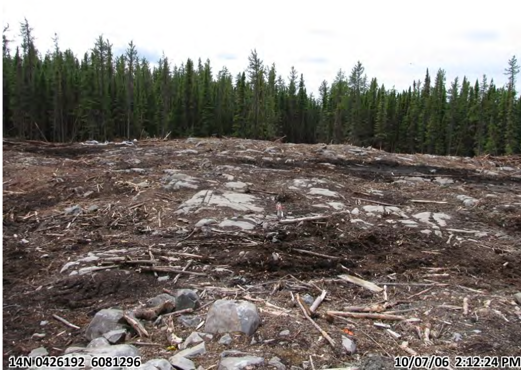
Photograph 15. Panoramic of cleared Lalor site, numerous bedrock ridges (6 July 2010)
