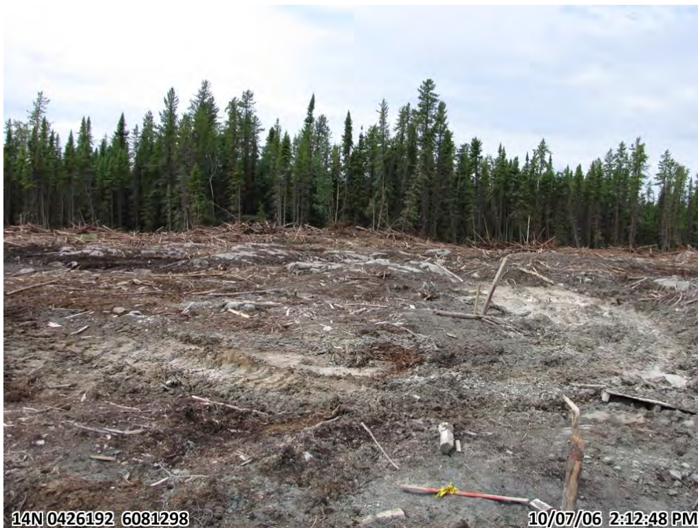
Photograph 17. Panoramic of cleared Lalor site, numerous bedrock ridges (6 July 2010)
