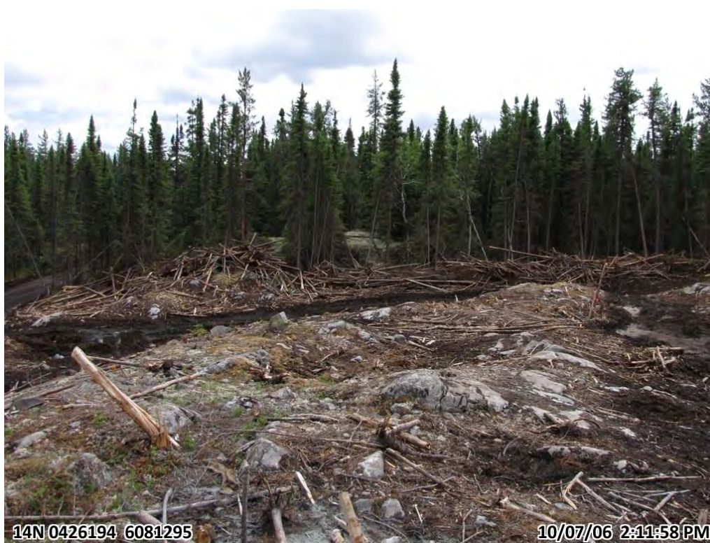
Photograph 13. Panoramic of cleared Lalor site, numerous bedrock ridges (6 July 2010)
