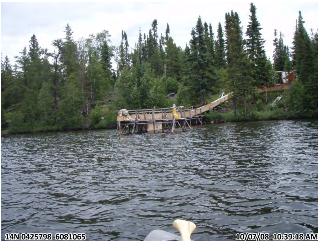
Photograph 01. Lalor Lake temporary water supply (8 July 2010)
