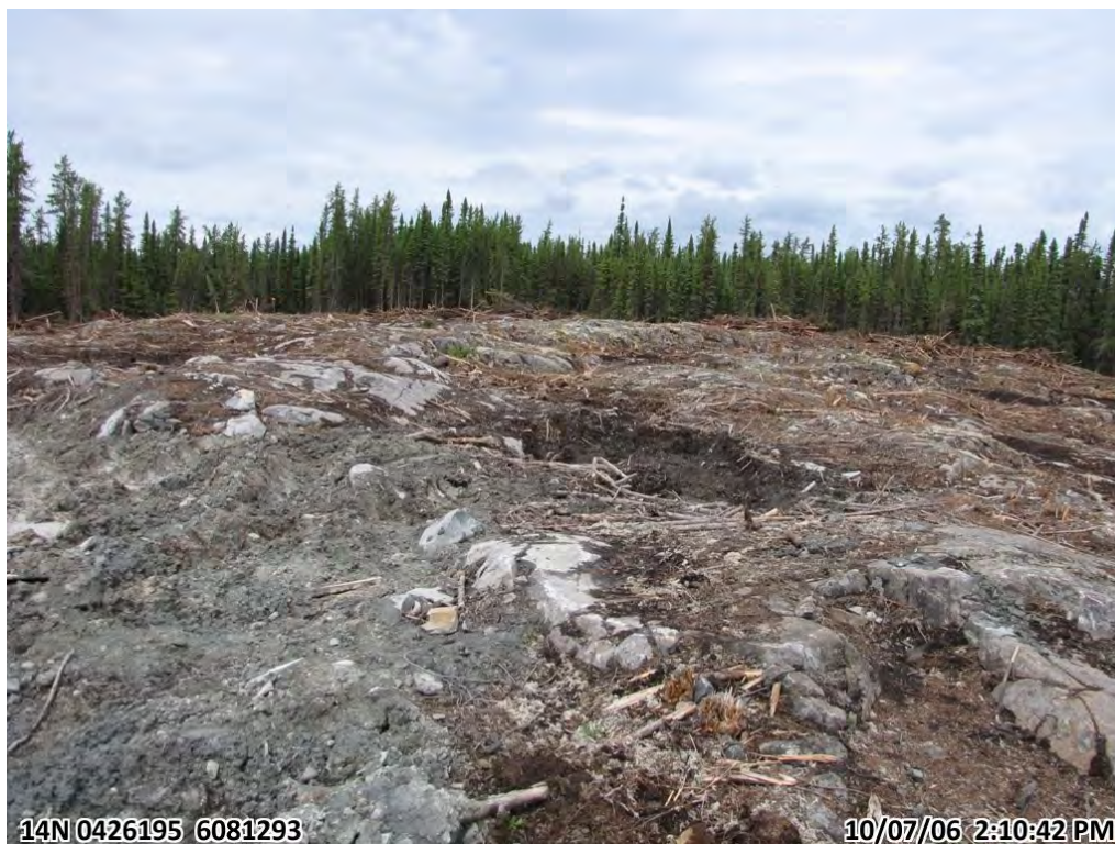
Photograph 08. Panoramic of cleared Lalor site, numerous bedrock ridges (6 July 2010)
