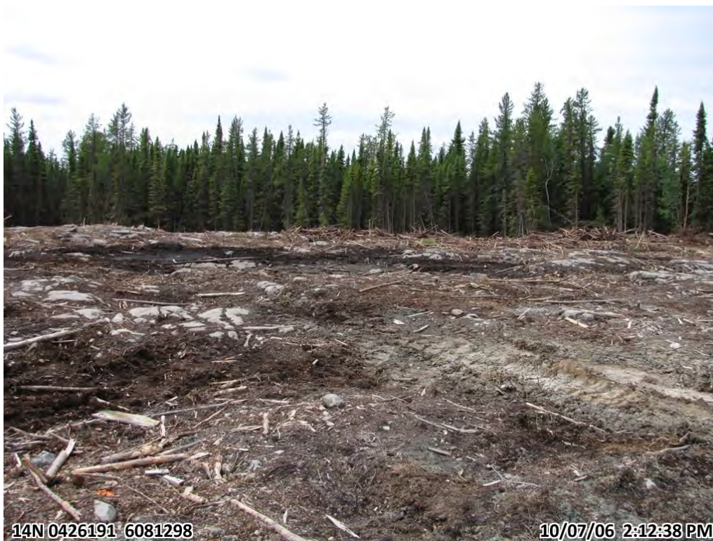
Photograph 16. Panoramic of cleared Lalor site, numerous bedrock ridges (6 July 2010)
