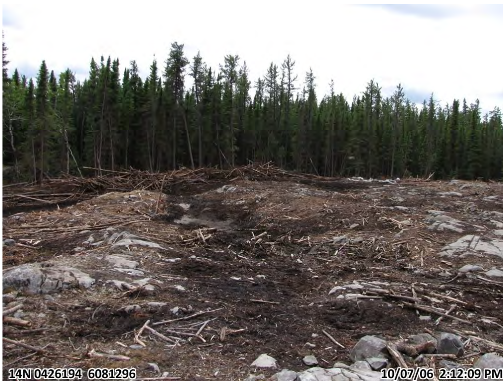
Photograph 14. Panoramic of cleared Lalor site, numerous bedrock ridges (6 July 2010)
