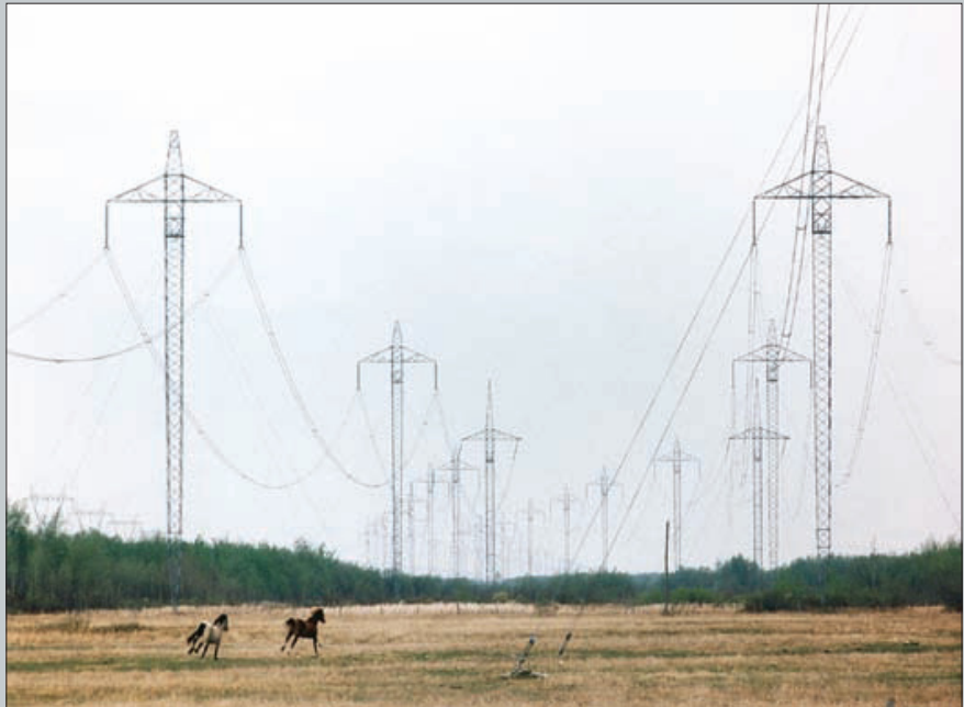
An HVDC line in Manitoba
