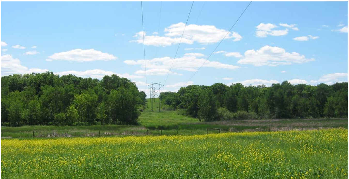
Special management practices are identified for every transmission line project
