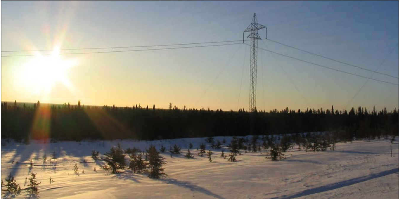
A transmission line in northern Manitoba
