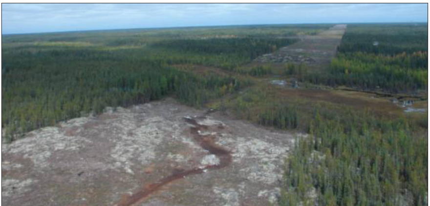
A buffer zone is established at a stream crossing
