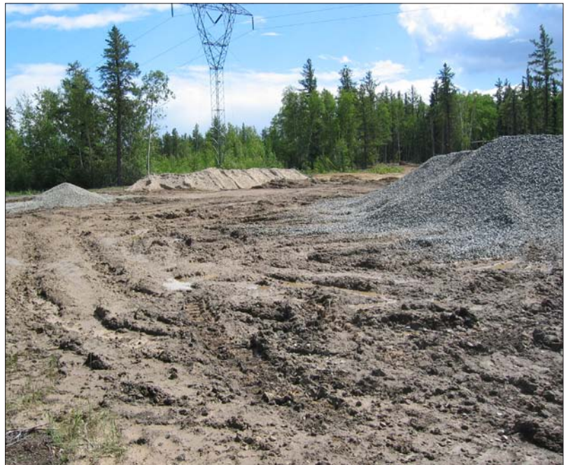
Borrow pits are areas where fill materials such as gravel, sand, silt and clay are excavated for use in foundation construction
