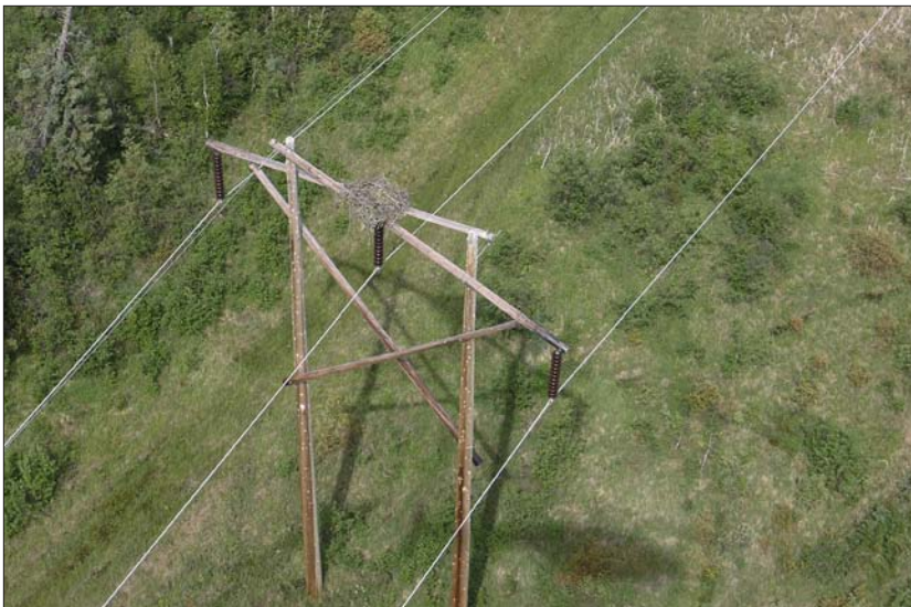
An osprey nest on a transmission line structure
