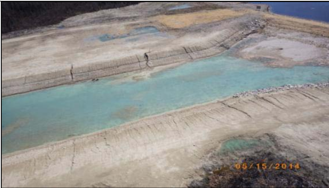
Figure 17 Erosion along Reach 1
