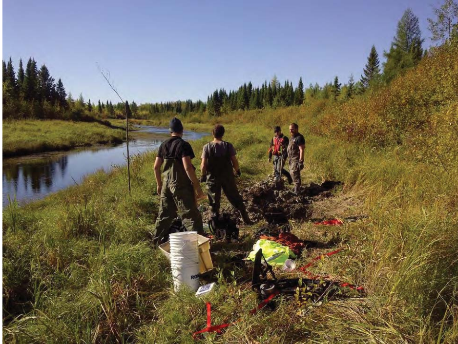
Photo 7 – View of work area
