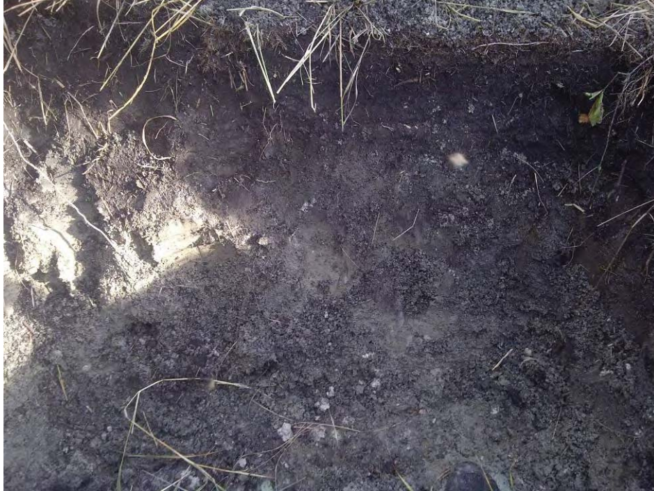
Photo 1 – Side wall of testpit
