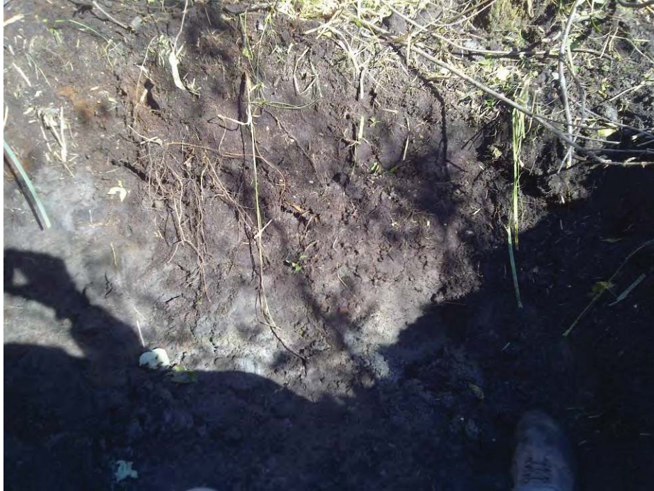
Photo 1 – Side wall of testpit
