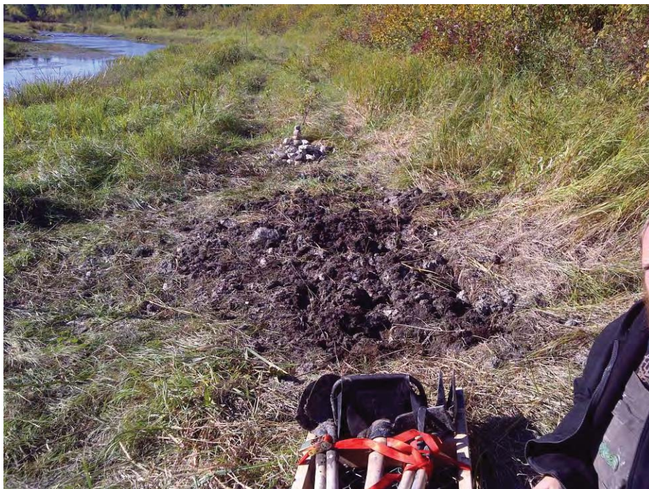
Photo 8 – Testpit backfilled
