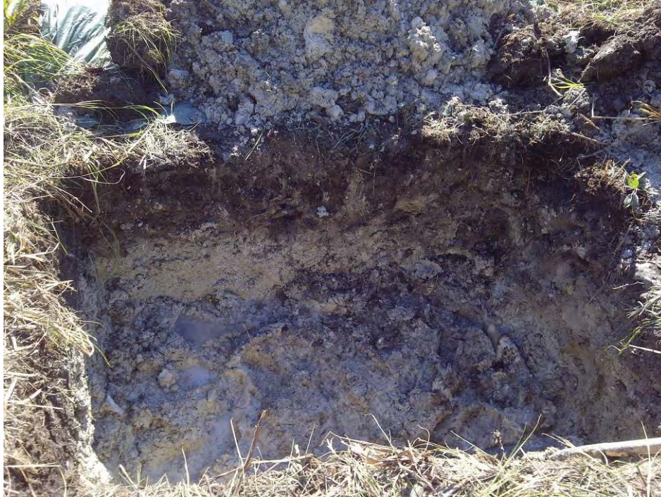
Photo 1 – Side view of testpit
