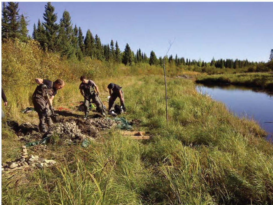
Photo 6 – Backfilling testpit
