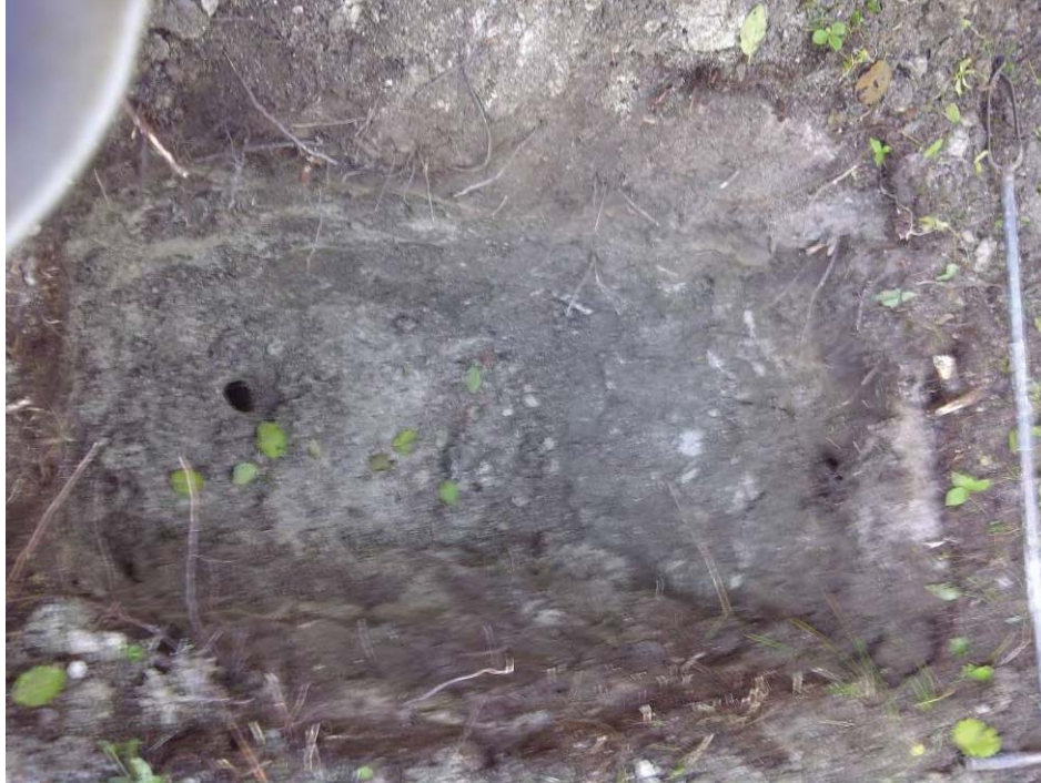
Photo 1 – Base of testpit
