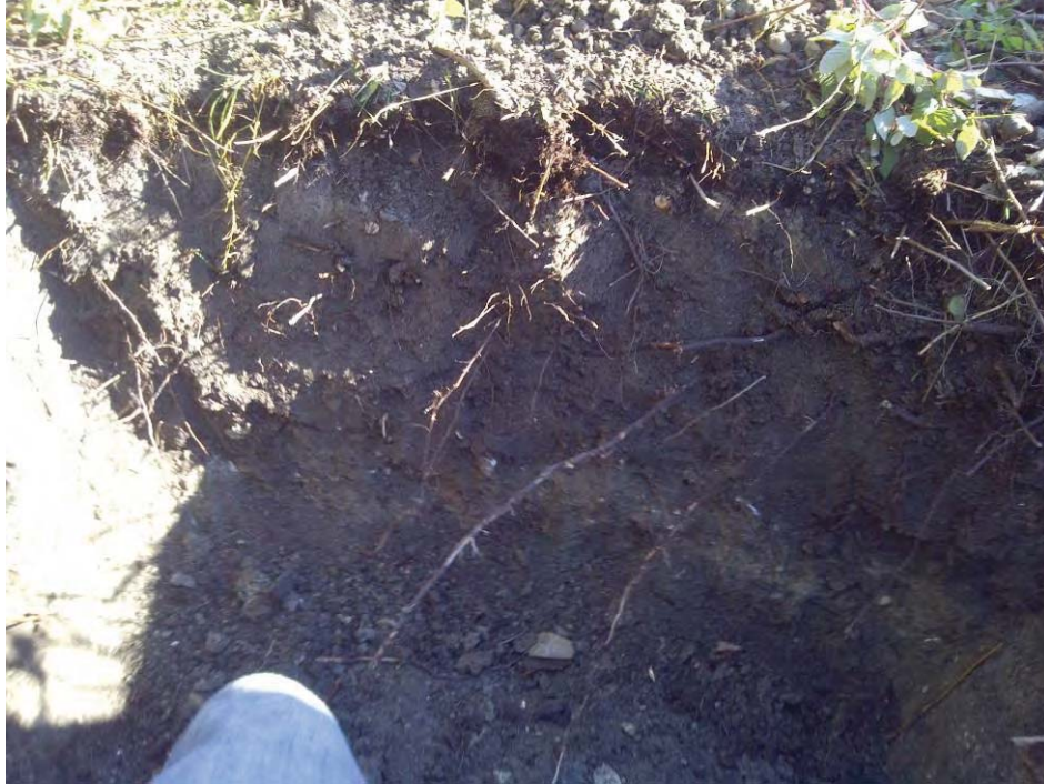
Photo 1 – Side wall of testpit
