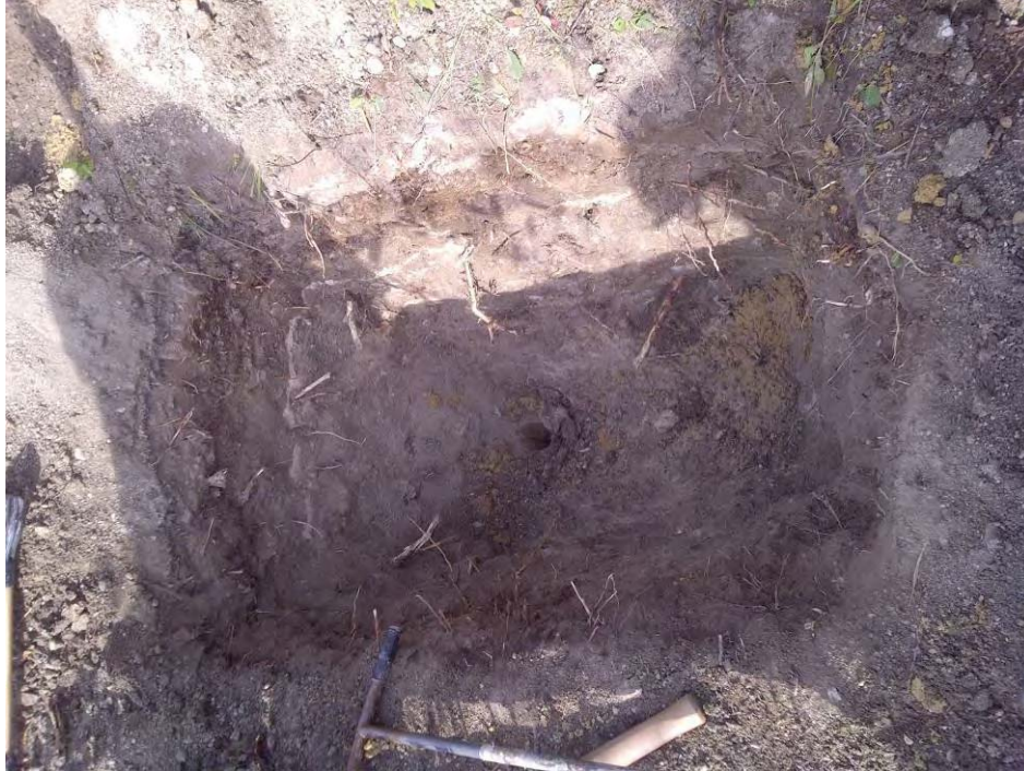
Photo 3 – Base of testpit showing auger hole
