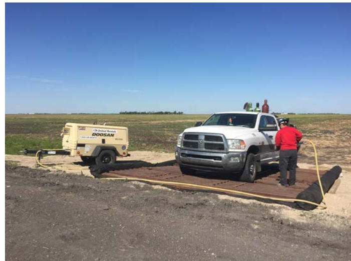
Compressed Air Cleaning Station at Controlled Access point
