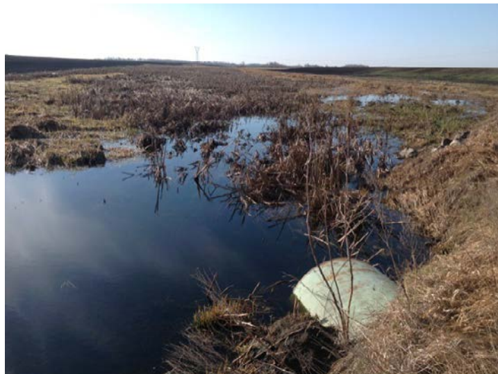
Figure 5-1 Ephemeral drain at southern end of route
