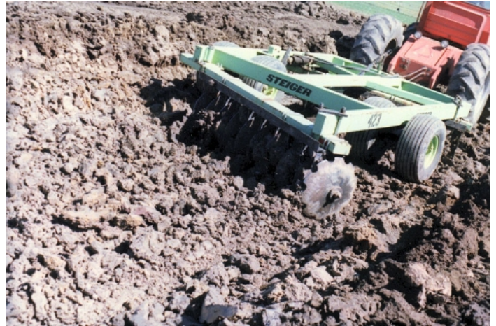
Heavy duty offset disc harrows may be used to scarify soil between lifts placement.
