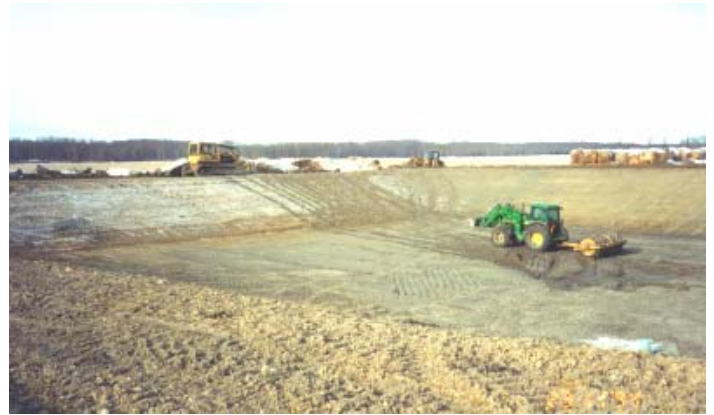
Depending on the site hydrogeology, an earthen manure storage may require a compacted clay liner.
