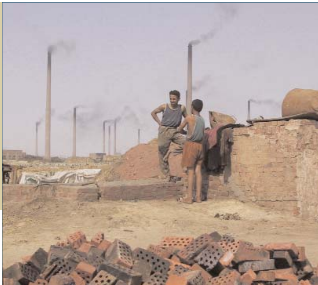
▲ Roche Consulting, in a joint project with CIDA, helped 50 brick factories in the Egyptian province of Arab Abu Saed to convert from oil to natural gas in an effort to reduce greenhouse gas emissions, representing 100,000 tons of emissions per year. Other benefits of this project included technology transfer, environmental awareness training and a better quality of life for workers and villagers.
