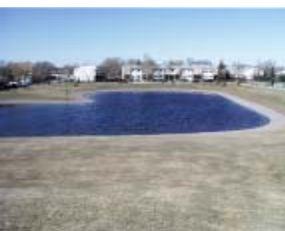
Below: A stormwater retention pond.
