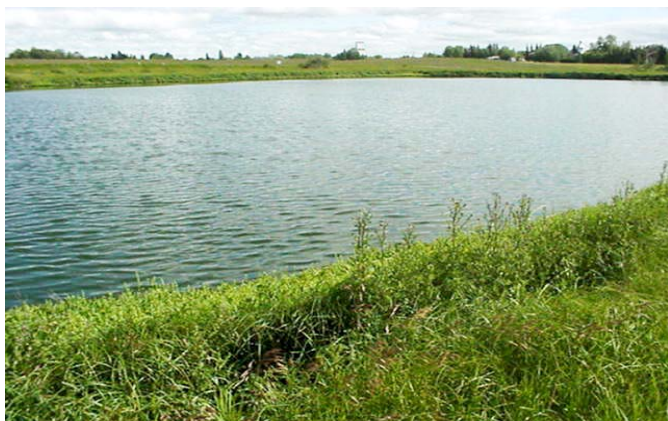
A typical municipal sewage lagoon.
