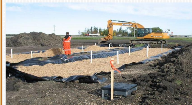
Woodchip bioreactor being researched at Agriculture and Agri-Food Canada, Morden
