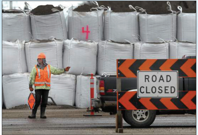
Superbags are used in areas where there is sufficient access .
