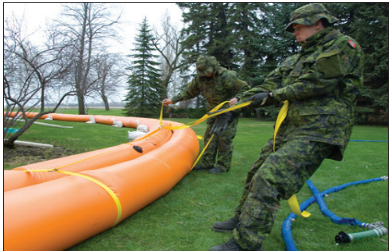
Aqua Dams and Tiger Dams are effective against shallow, overland flooding.
