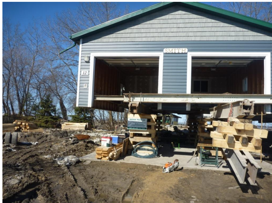
Raising permanent dwelling to higher elevation
