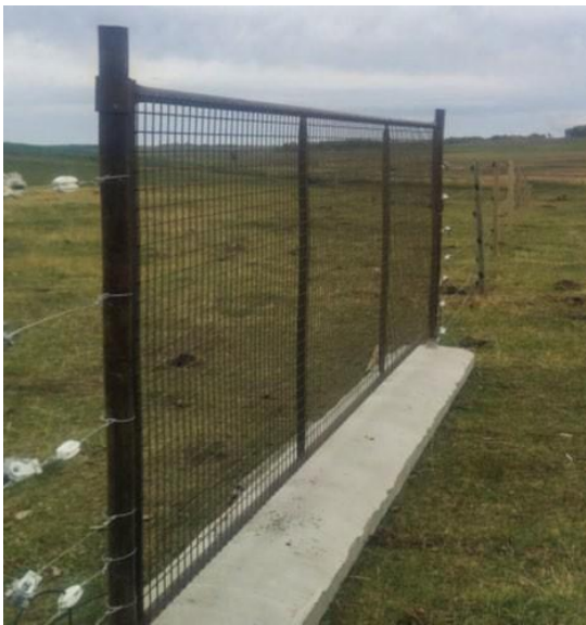
Gate with concrete threshold
