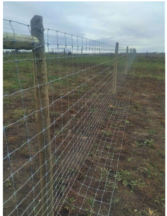
Fixed-knot fence with apron to deter burrowing
