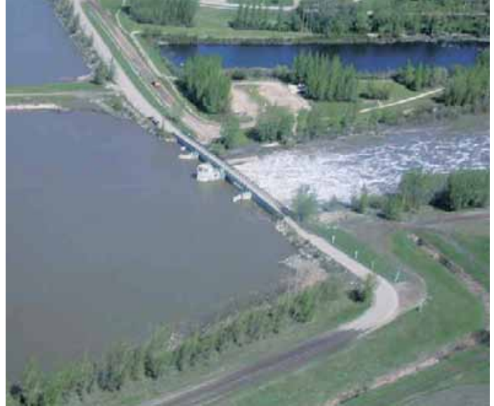
Portage Diversion structure
