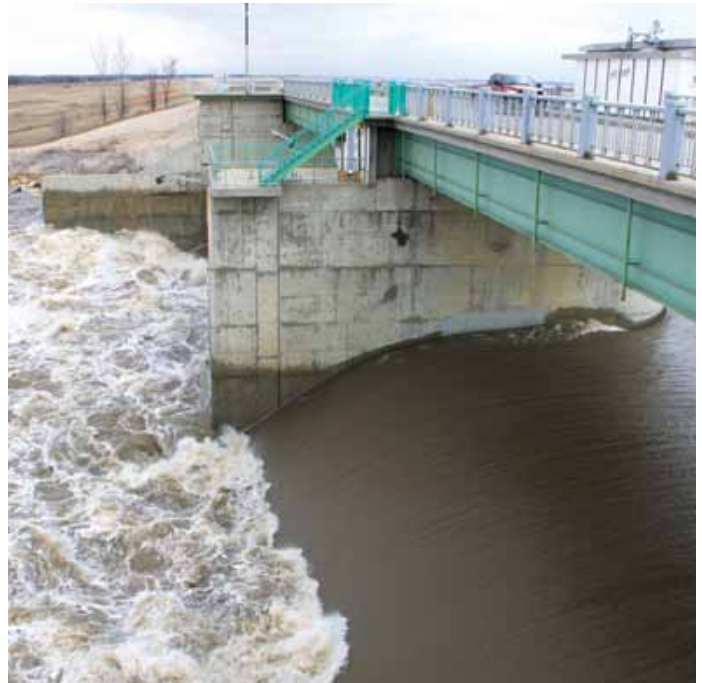
Floodway inlet control structure south of Winnipeg
