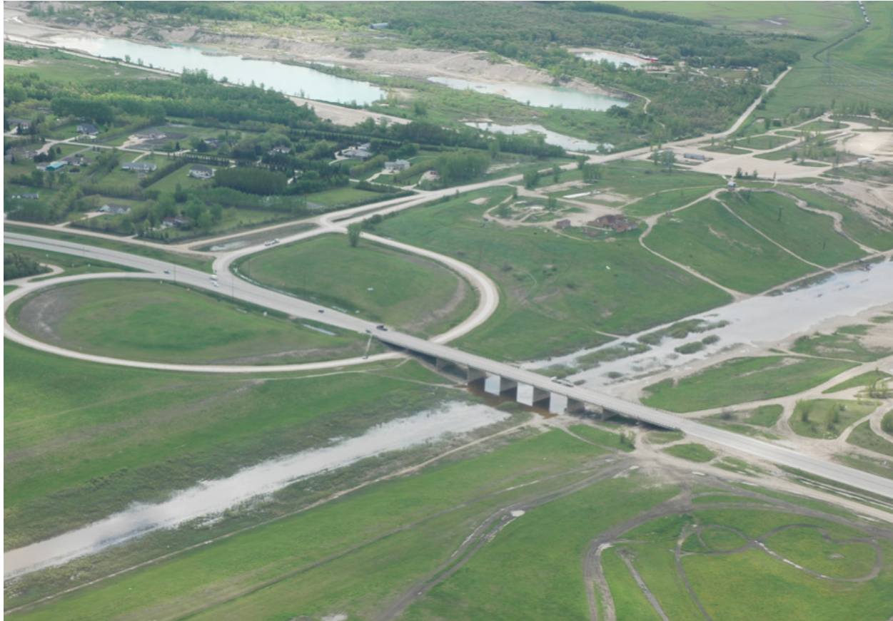
Figure 4.6-15 Aerial View of the Existing PTH 59 Bridge Crossing Configuration
