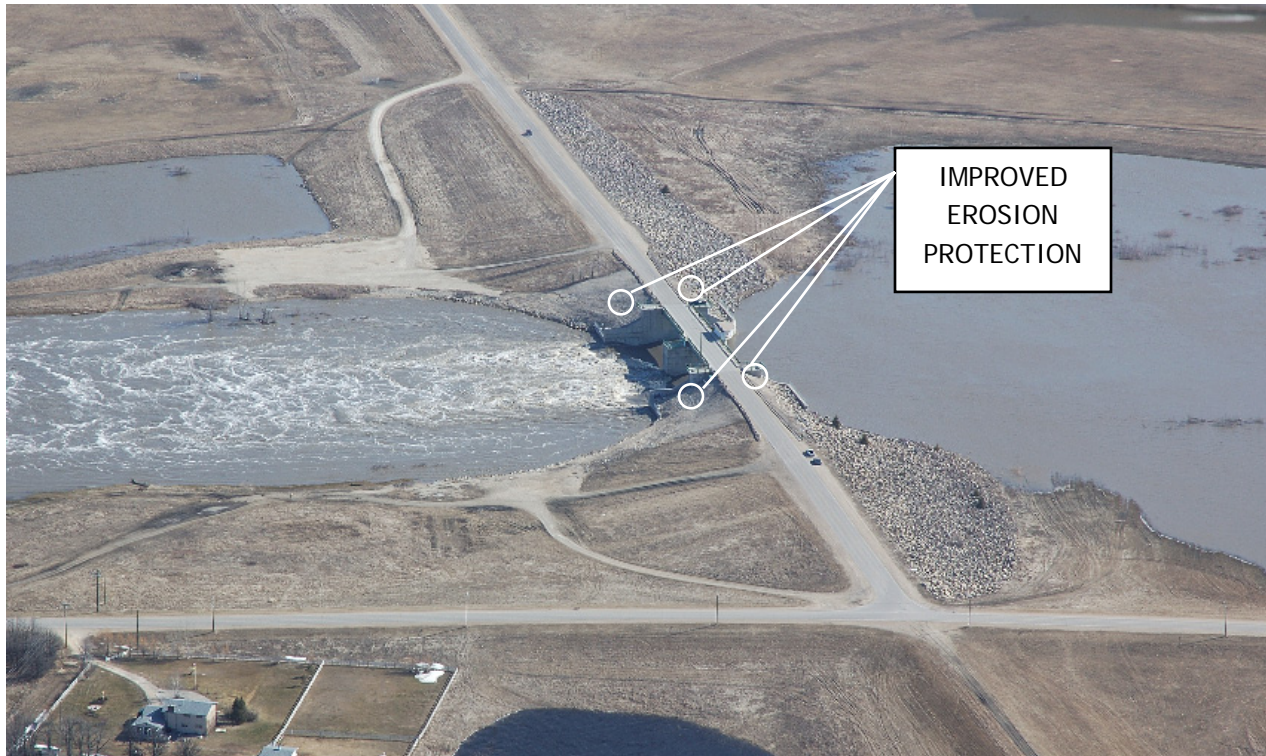
Figure 4.4-4 Floodway Inlet Control Structure and Earthfill embankments view from the west side of the Red River
