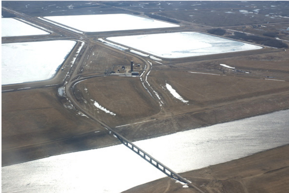
Figure 4-6.28 Existing GWWD Rail Bridge
