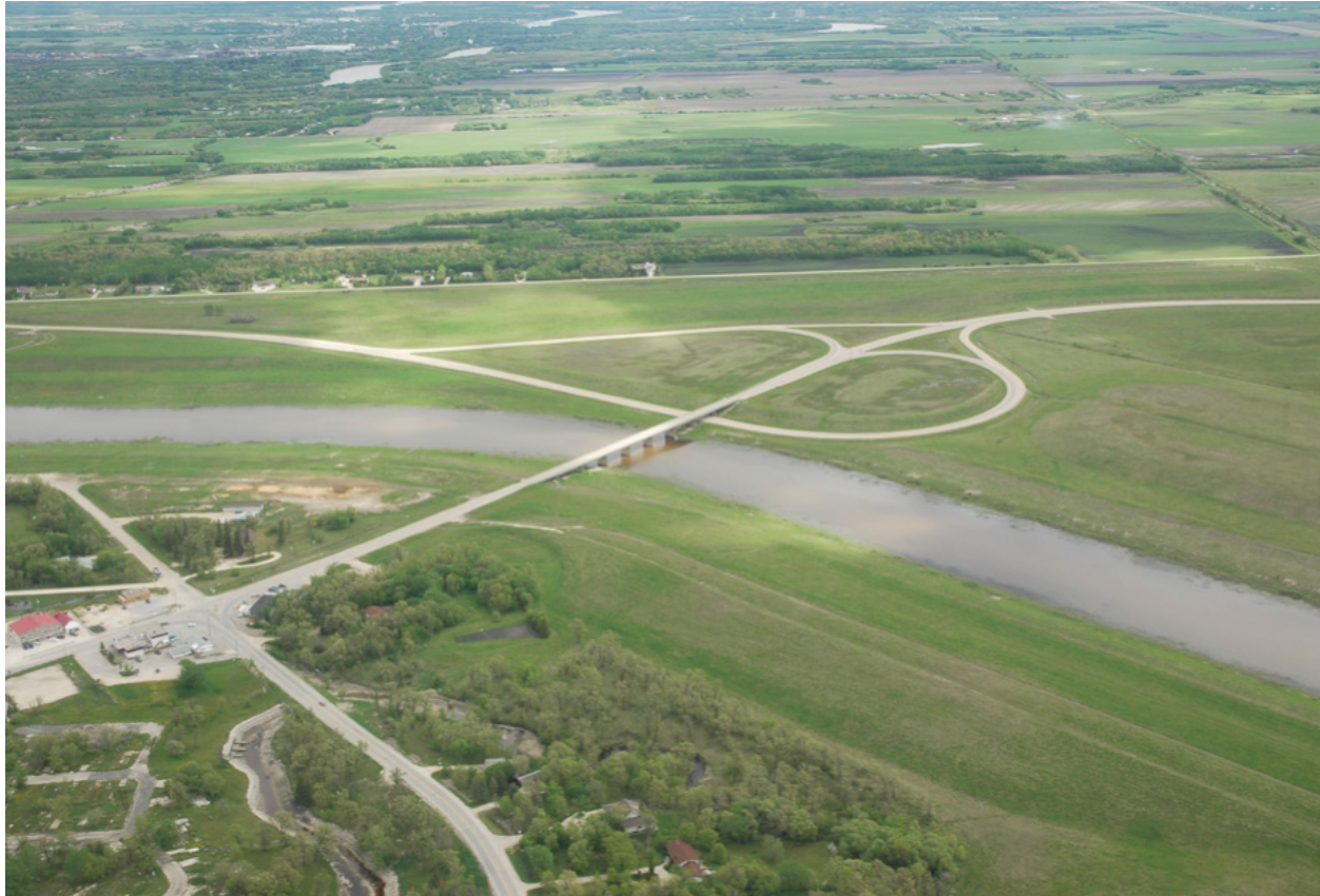
Figure 4.6-18 Aerial View of the Existing PTH 44 Crossing Configuration
