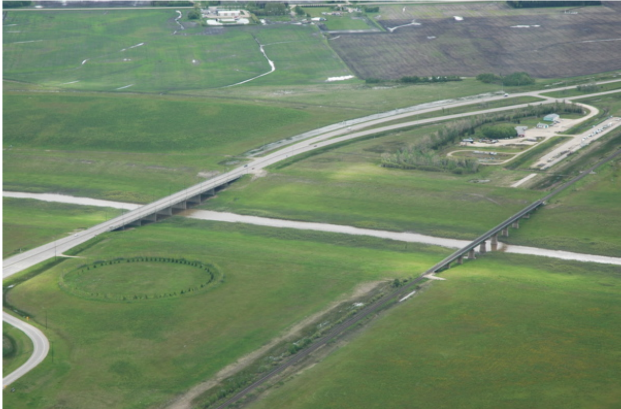
Figure 4-6.25 Existing CNR Sprague rail crossing.
