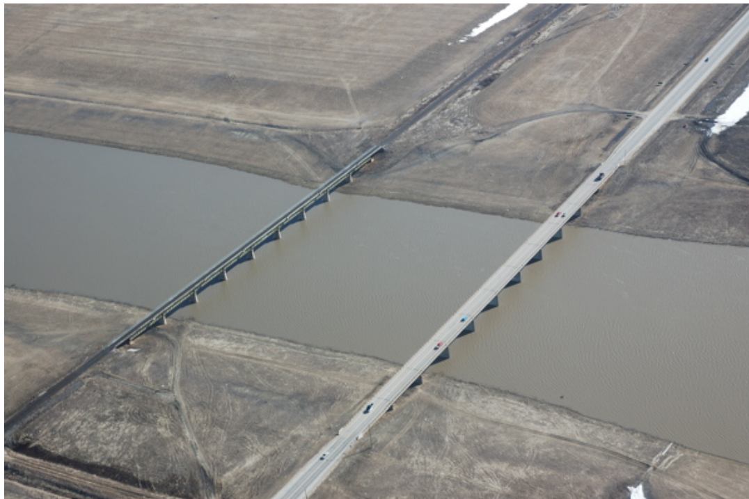
Figure 4.6-31 Existing CNR Redditt Rail Crossing (shown at left)
