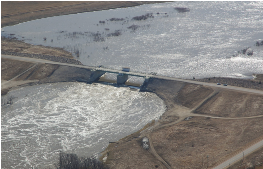
Figure 4.4-3 Floodway Inlet Control Structure and earthfill embankments as viewed from the north face upstream on the Red River
