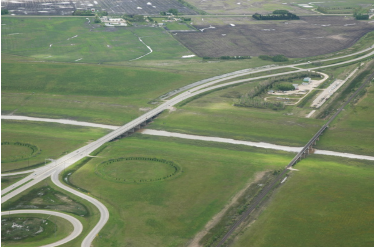
Figure 4.6-7 Aerial View of the Existing TCH No. 1 East Crossing
