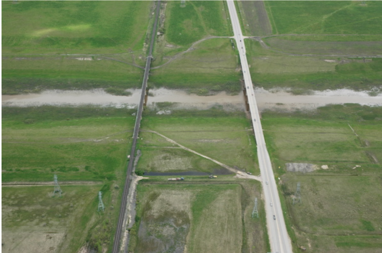
Figure 4-6.12 Aerial View of the Existing PTH 15 Highway Bridge Structure
