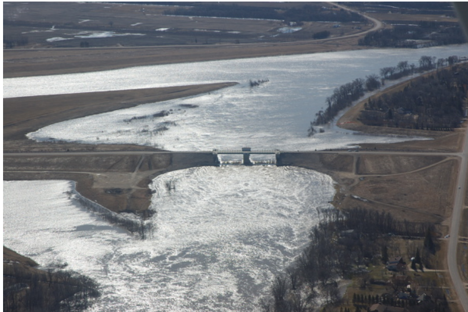
Figure 4.4-1 Aerial view of Inlet Control Structure looking upstream along the Red River. The Floodway is shown in operation during April 2004 spring flooding. Floodway channel is in background.
