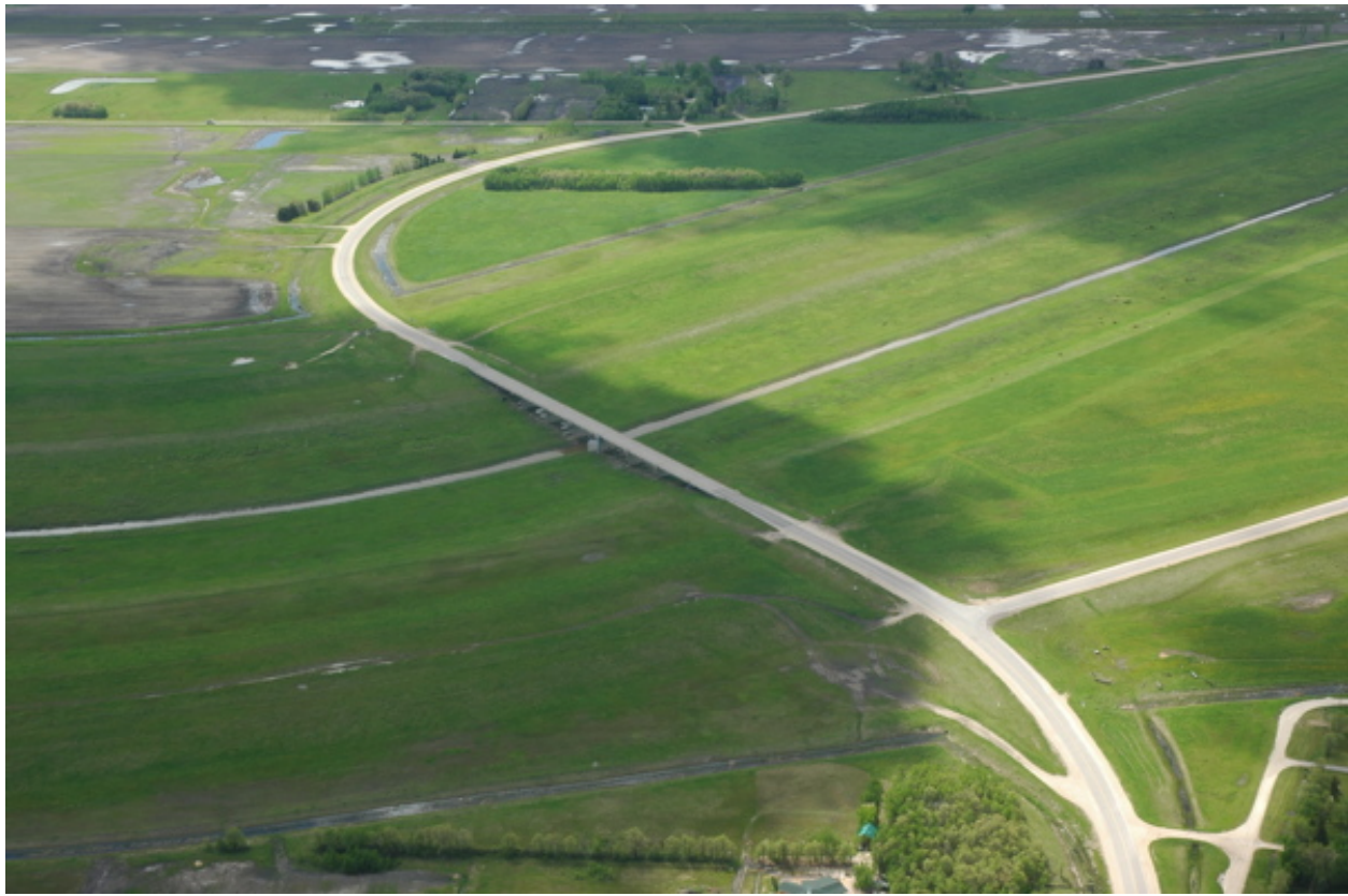
Figure 4.6-1 St. Mary's Road PR 200 Highway Bridge Crossing
