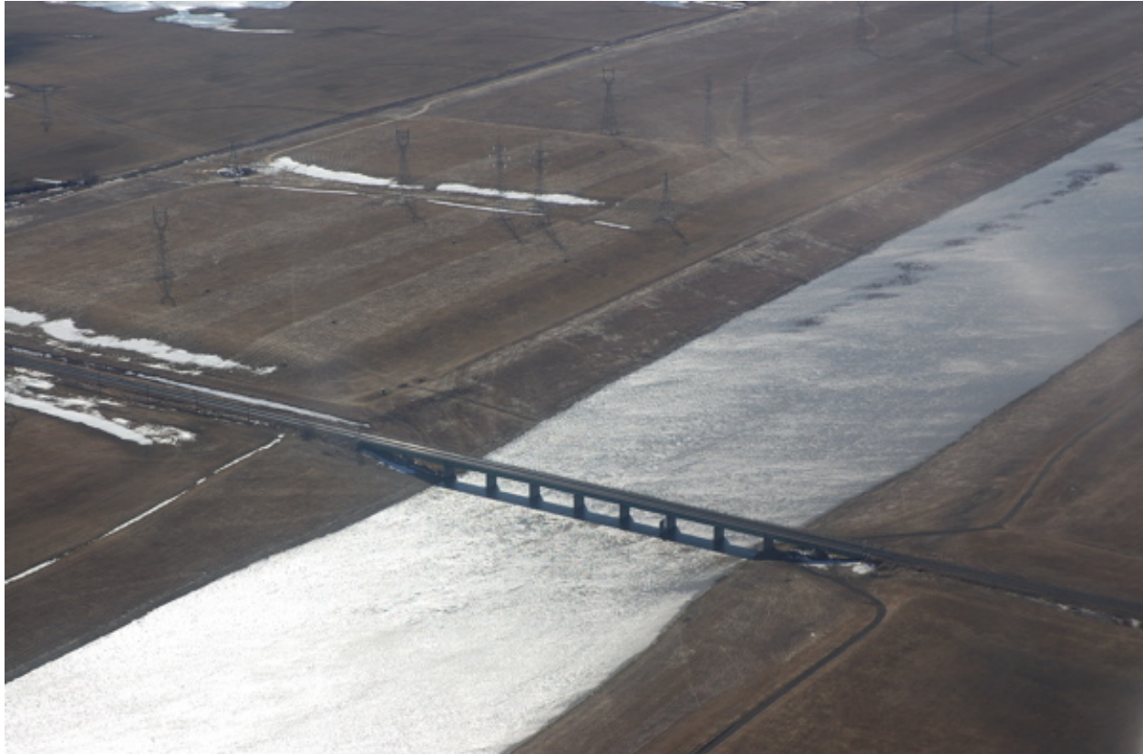
Figure 4.6-34 Existing CPR Keewatin Rail Crossing.
