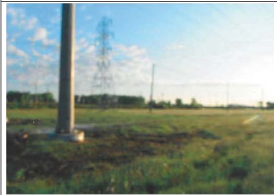
Photo 11: PL-4; looking N at Hydro tower GPS Location: Northing 5523409, Easting 631780
