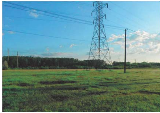
Photo 14: PL-5; looking N at Lattice Hydro tower GPS Location: Northing 5523292, Easting 631561
