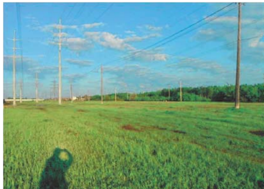
Photo 15: PL-5; looking W at distribution poles GPS Location: Northing 5523292, Easting 631561
