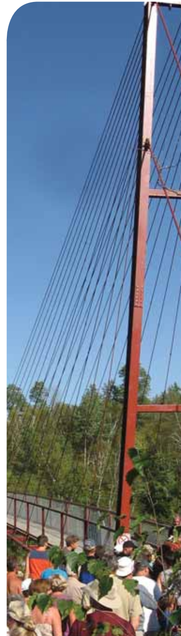
▲ Whiteshell River Bridge, Manitoba.
