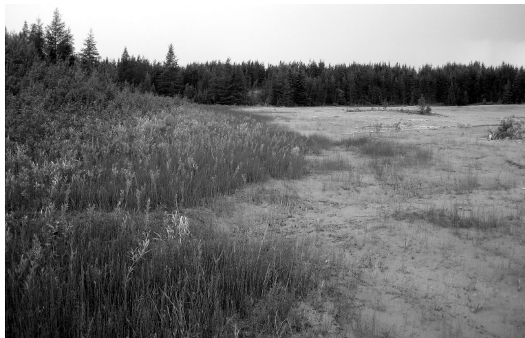
Figure GS-12-1: Gunnar mine tailings site; south side (on the left) covered with vegetation and north side (on the right) with very limited vegetation.
