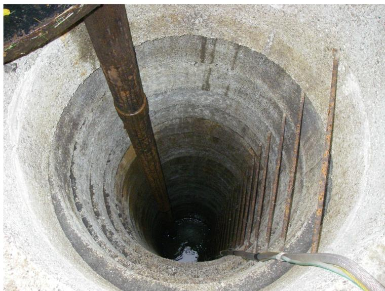
**Figure GS-18-2:** Old hand-dug well near Notre Dame de Lourdes at SE-30-7-8-W1 with visible bubbles at the water-table surface; pipe on the left side captures gas and is flared occasionally for short periods of time. Well is approximately 1 m in diameter.
