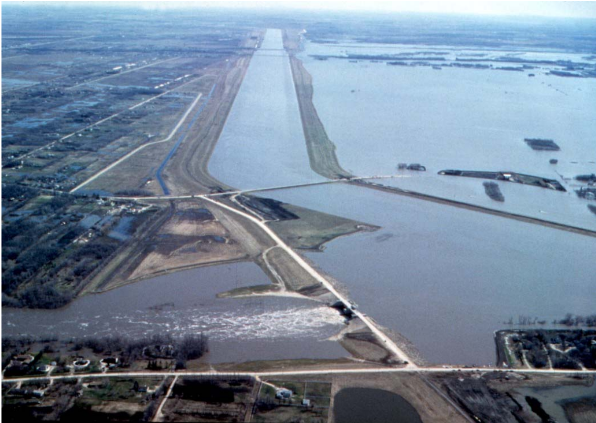
Figure 2: The Winnipeg floodway narrowly contained flood flows in 1997. An additional rise of two feet would likely have overwhelmed Winnipeg's diking system and caused several billion dollars in damages.
